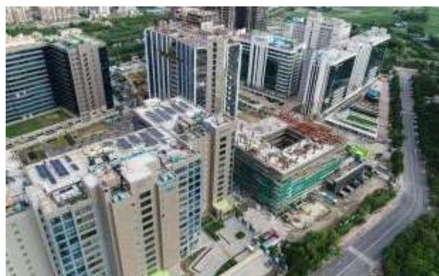
Tower 11 A (as of September 2020)
