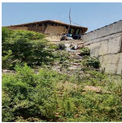
MNBR at Ch. 03+142
