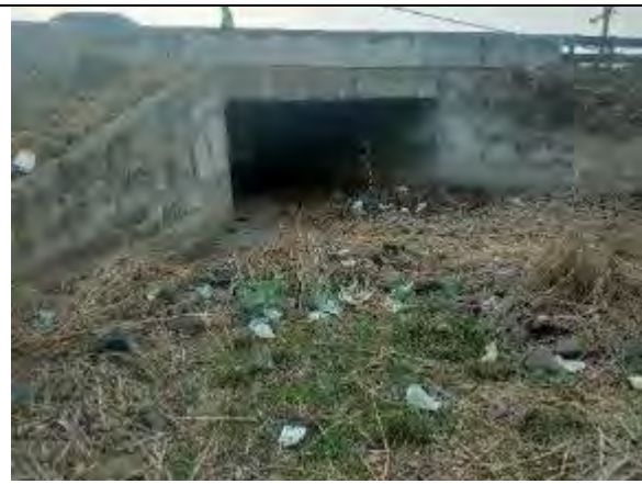
Box Culvert at Km 141+925
