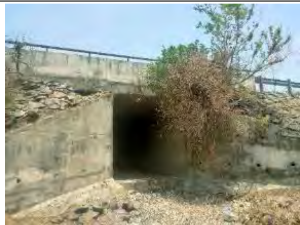
Box Culvert at Km 95+914
