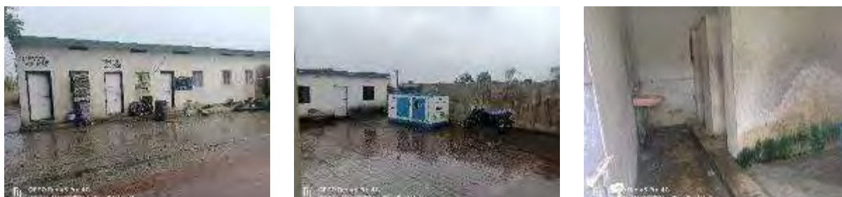
Figure 2-4. Facilities at Darodha Toll Plaza
