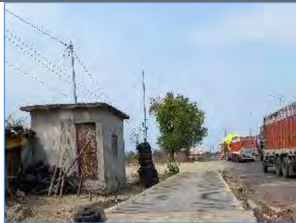
Weigh bridge, LHS @ 92+500
