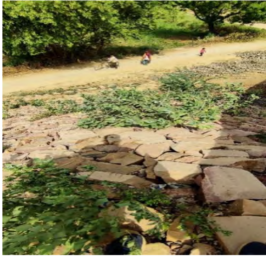
MNBR at CH. 17+661
