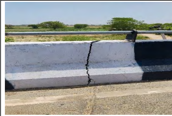
MNBR at CH.1+838
