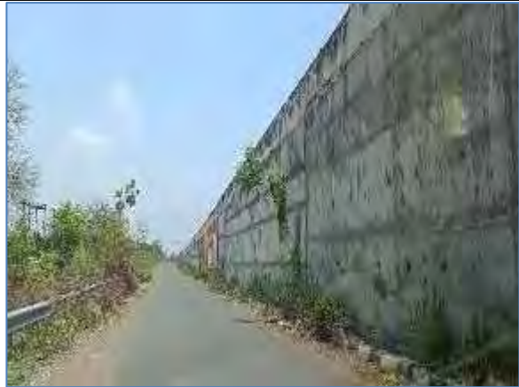
Service Road @ km 66.700 to km 67.350-LHS_5.5m wide
