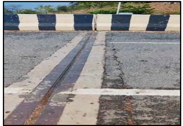
Major Bridge at Ch. 1319+870
