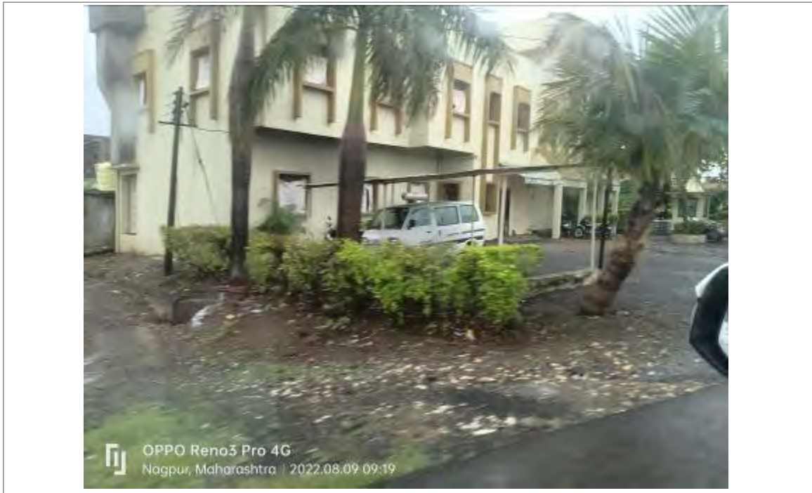
Photo 1: Toll plaza building
