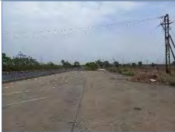
Truck Lay bye on LHS km 68.240
