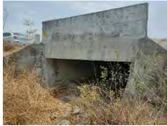
Slab Culvert at Km 45+985
