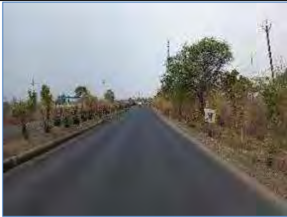
Fair condition km 88.000-LHS
