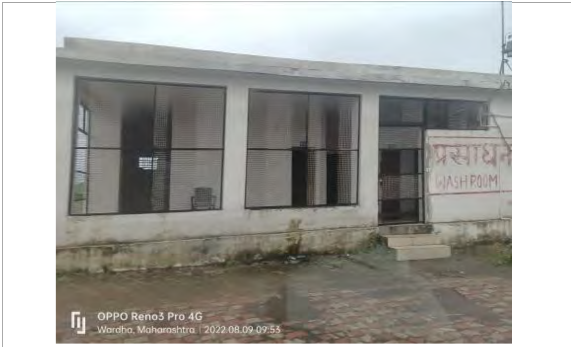
Photo 7: Washroom facility on the toll plaza
