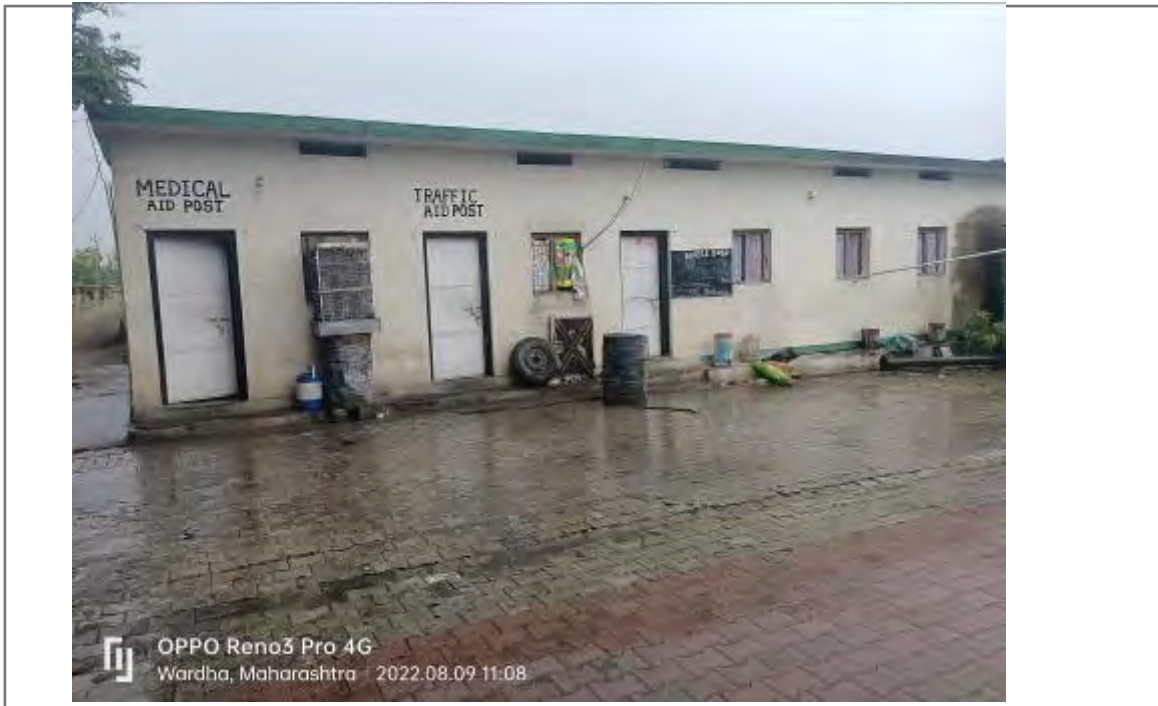
Photo 12: Medical aid post and traffic aid post facility at toll plaza
