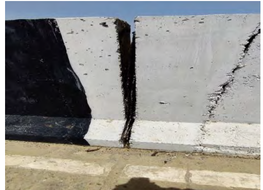
ROB at CH 8+954
