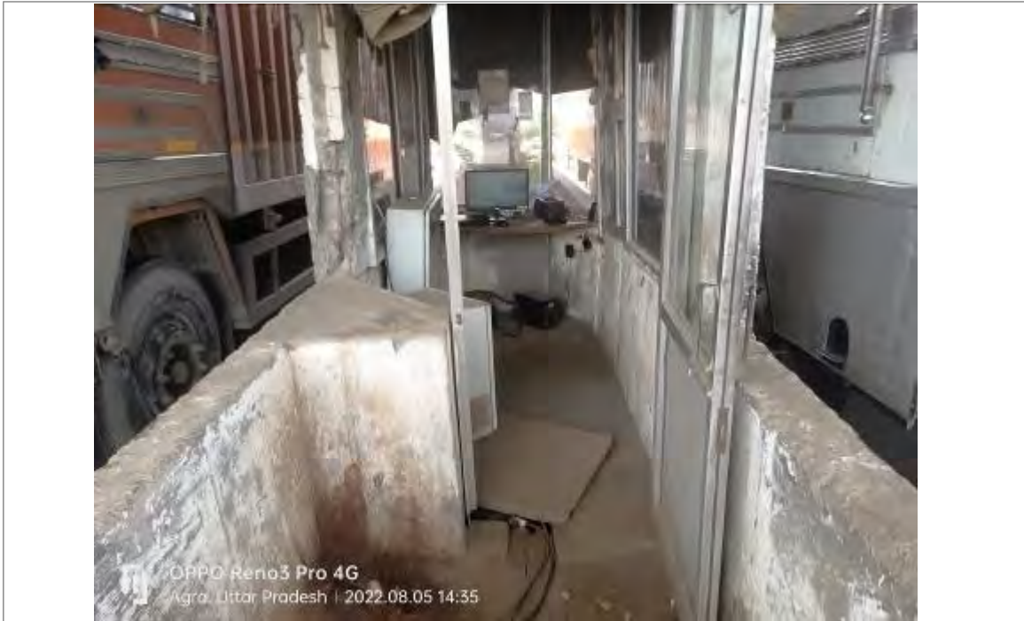
Photo 9: Inside view of toll booth
