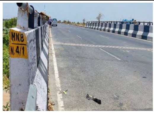
MNBR at CH. 3+142
