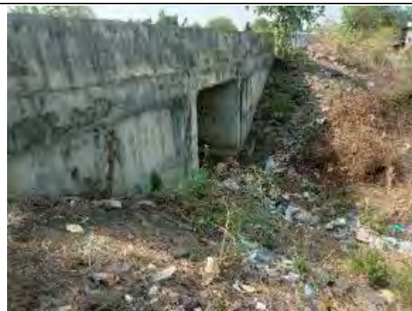
Box Culvert at Km 134+395
