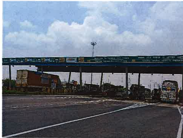
Raibha Toll Plaza
