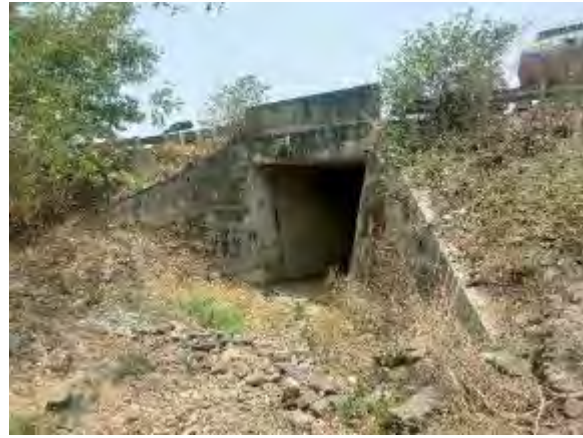
Slab Culvert at Km 42+335
