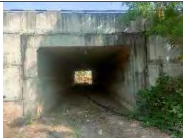
Box Culvert at Km 66+244
