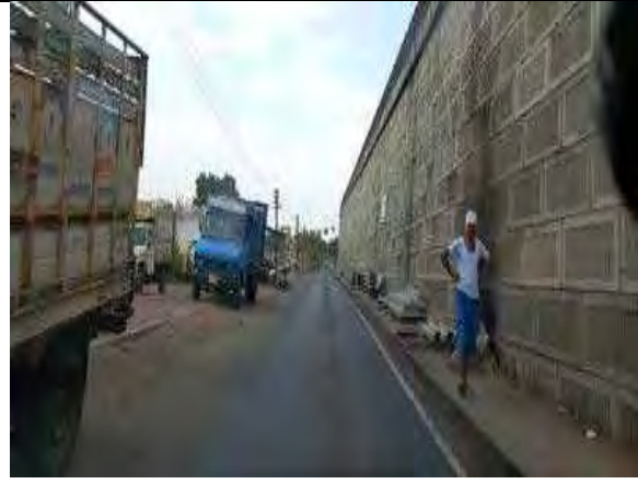
Service Road @ km 132.320 to km 134.080-RHS_6m wide
