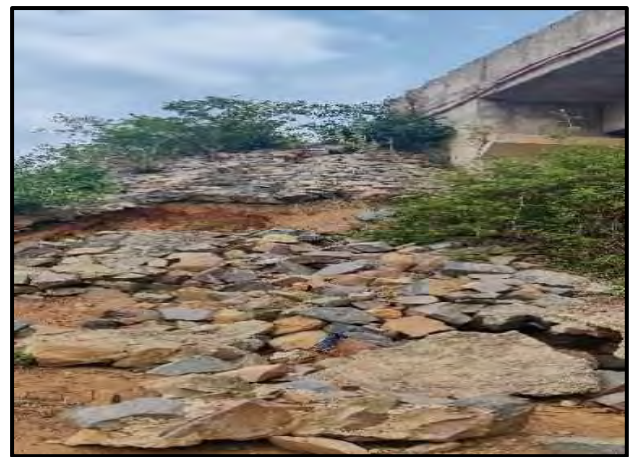
Major Bridge at Ch. 1356+285
