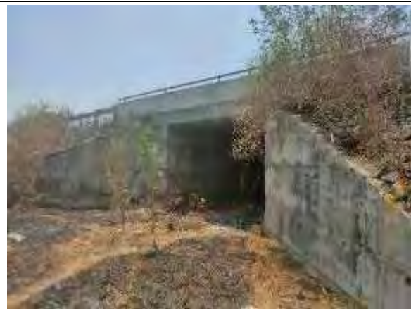
Box Culvert at Km 93+985
