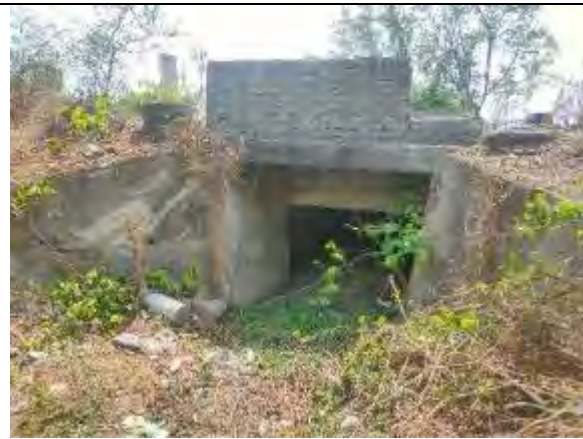
Slab Culvert at Km 51+180
