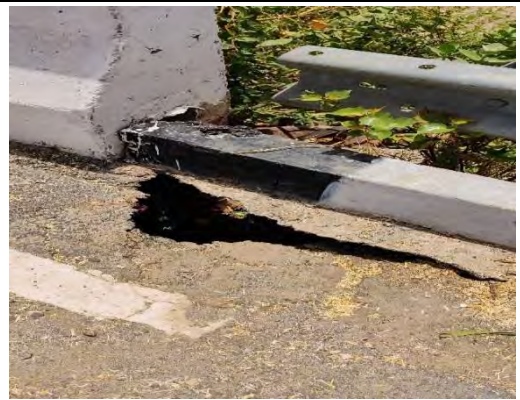
MNBR at CH 6+799
