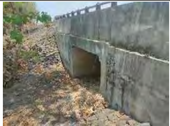
Box Culvert at Km 161+580
