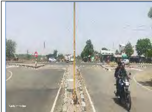
Major Junction at km 59.457 LHS
