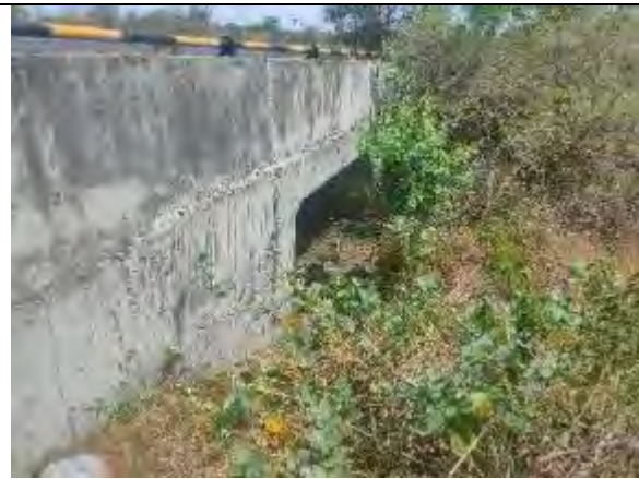
Box Culvert at Km 83+092
