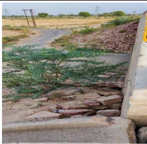
MNBR at Ch. 15+661
