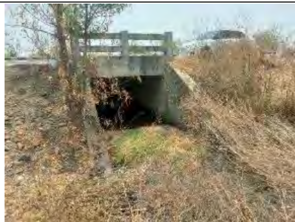
Slab Culvert at Km 46+847
