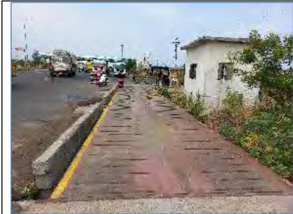
Weigh bridge, RHS @ 92+500
