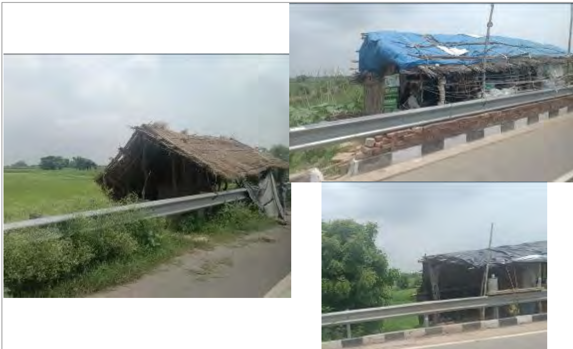
Photo 2: Encroachments in the ROW
