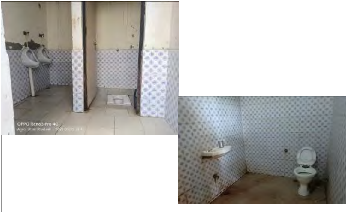
Photo 6: Toilet facilities at the toll plaza
