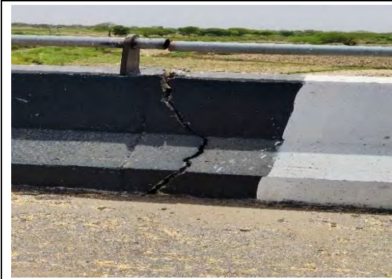
MNBR at CH.6+799
