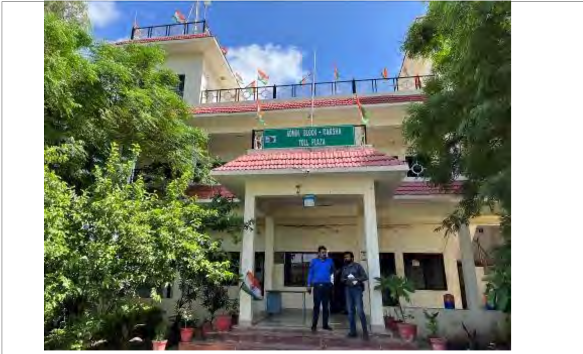
Photo 1: Toll plaza building
