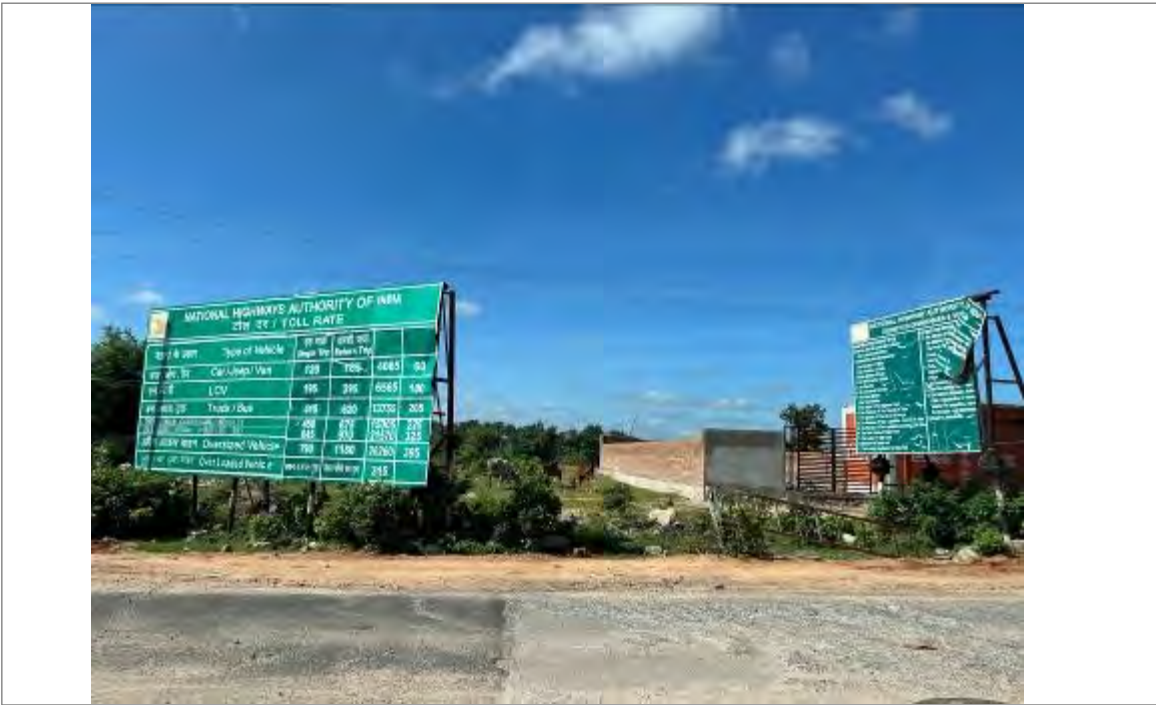
Photo 3: User Fee board and broken toll exemption board at the toll plaza
