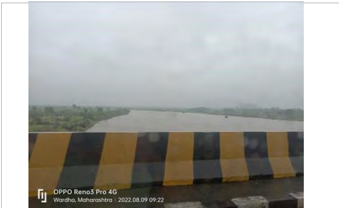
Photo 2: Bridge over the river in project area
