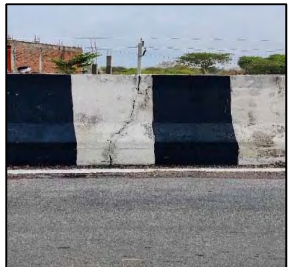
MINOR BRIDGE AT 1359+451
