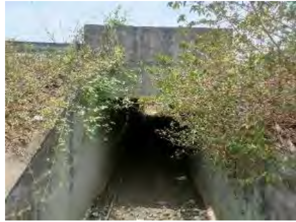
Box Culvert at Km 42+387
