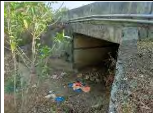
Box Culvert at Km 147+032
