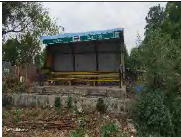
Bus shelter near km 153.090 on Service Road, LHS
