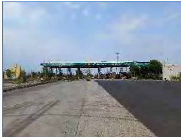
Toll Plaza at km 92+500
