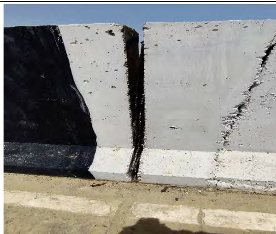
ROB at CH 8+954
