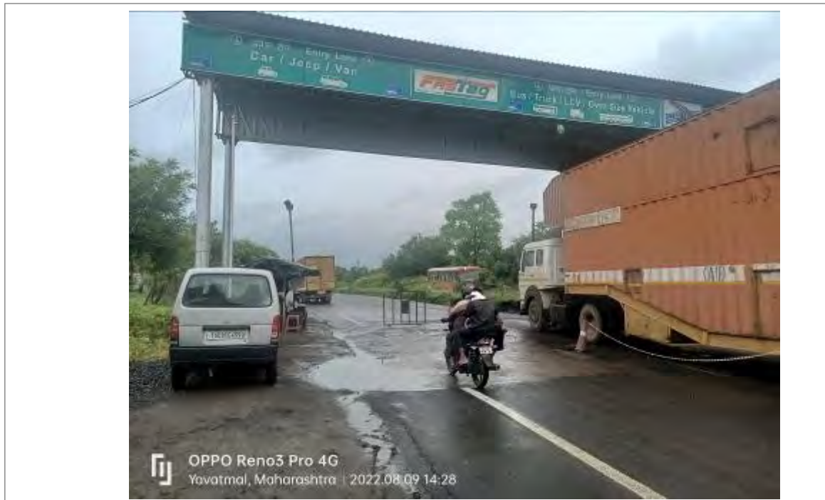
Photo 9: Electronic Toll Collection (ETC) lane
