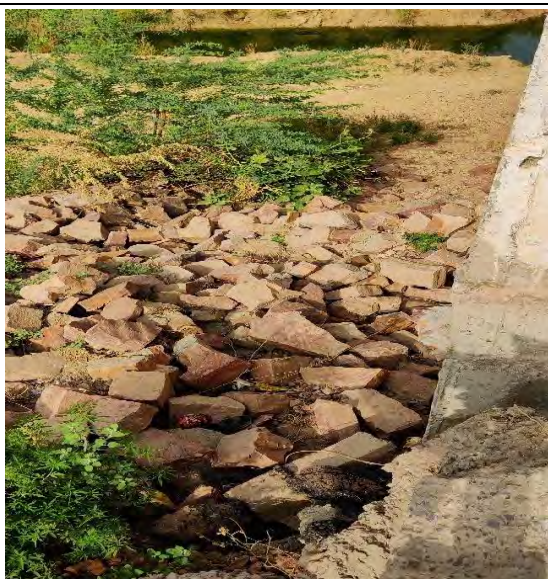
MNBR at CH. 31+547
