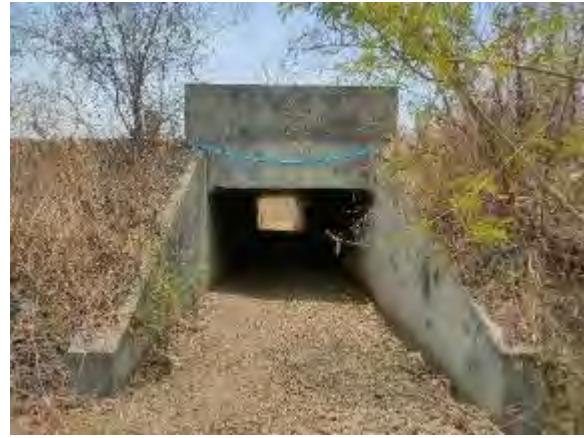
Box Culvert at Km 41+016
