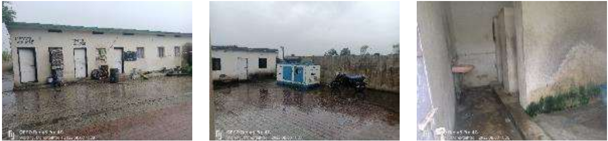
Figure 2-4. Facilities at Darodha Toll Plaza
