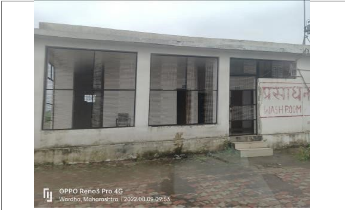
Photo 7: Washroom facility on the toll plaza
