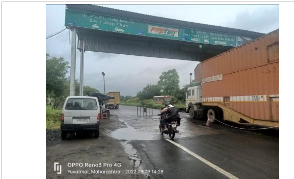
Photo 9: Electronic Toll Collection (ETC) lane
