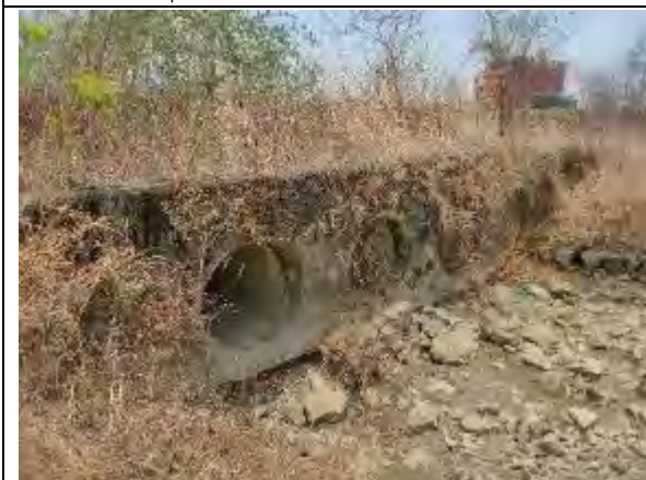
Pipe Culvert at Km 40+262
