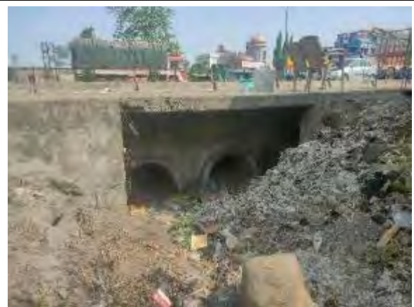
Pipe Culvert at Km 63+168
