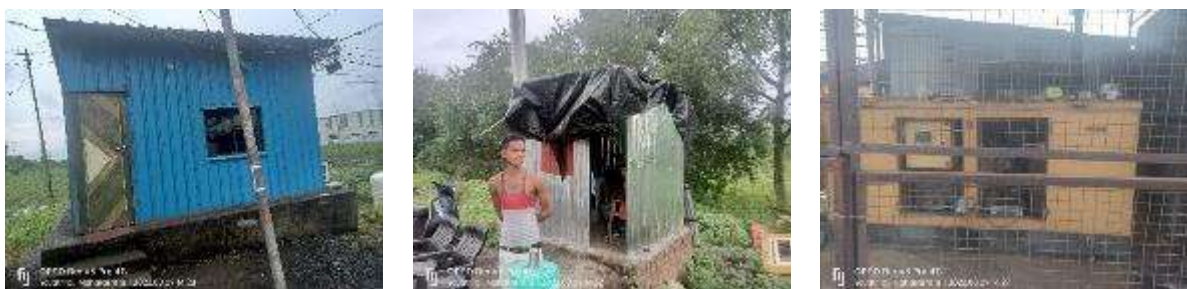
Figure 2-5. Kelapur Toll Plaza
