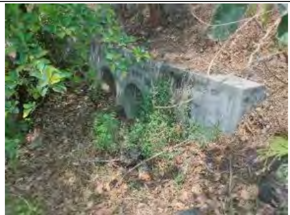
Pipe Culvert at Km 116+901
