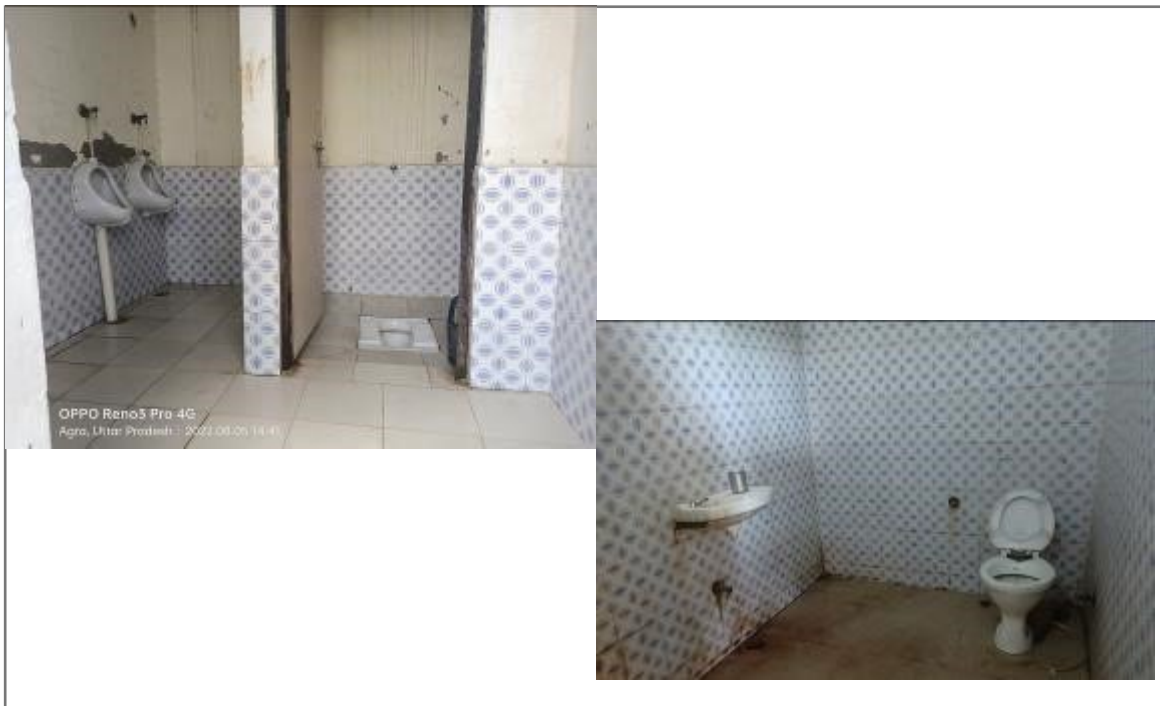
Photo 6: Toilet facilities at the toll plaza
