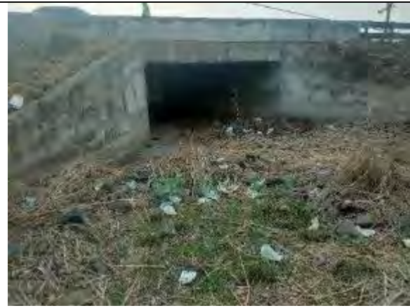
Box Culvert at Km 141+925
