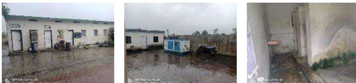
Figure 2-4. Facilities at Darodha Toll Plaza
