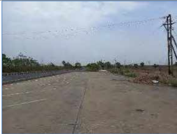
Truck Lay bye on LHS km 68.240
