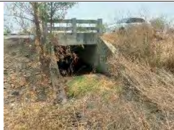
Slab Culvert at Km 46+847
