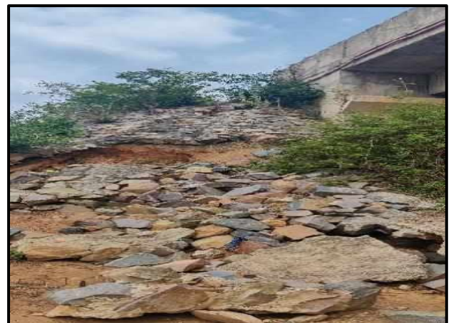
Major Bridge at Ch. 1356+285
