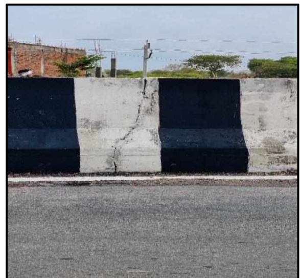
MINOR BRIDGE AT 1359+451
