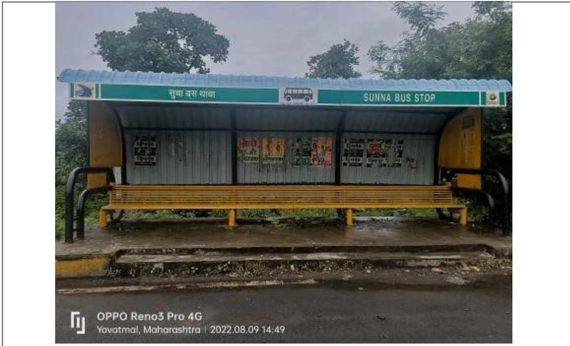
Photo 10: Bus stop along National highway
