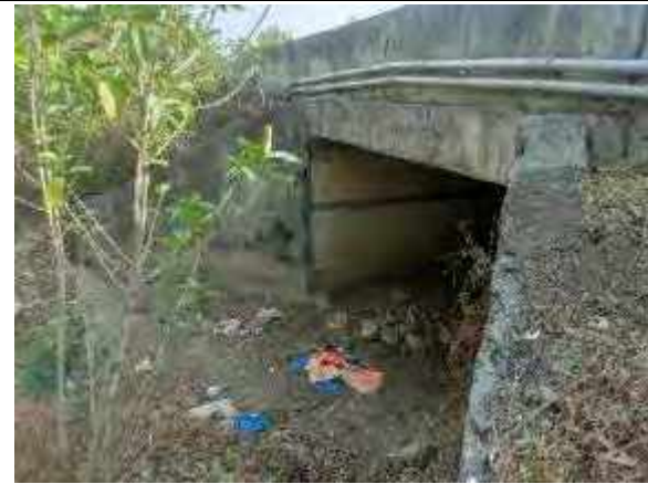
Box Culvert at Km 147+032
