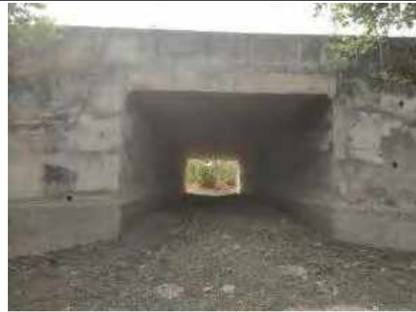
Box Culvert at Km 130+662
