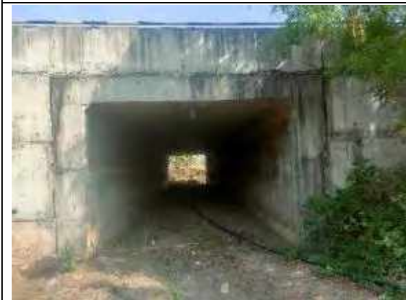
Box Culvert at Km 66+244
