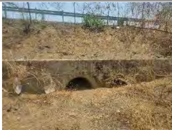
Pipe Culvert at Km 111+349
