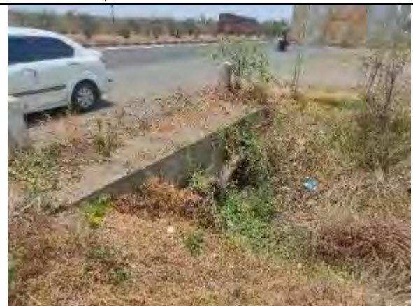
Pipe Culvert at Km 43+166
