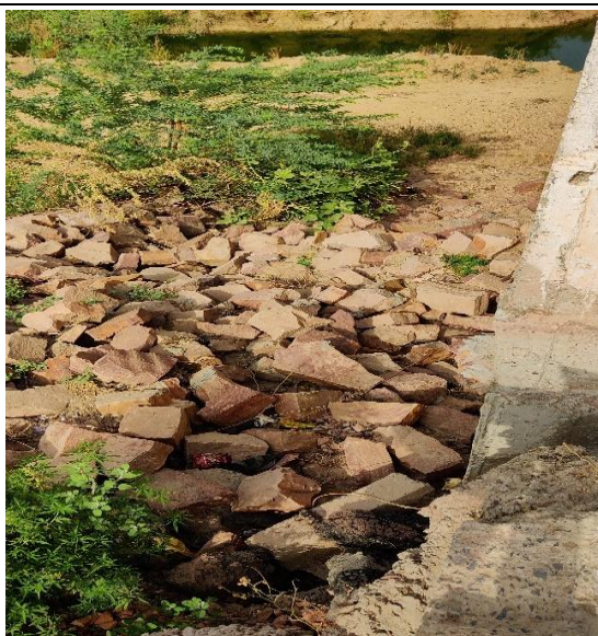
MNBR at CH. 31+547
