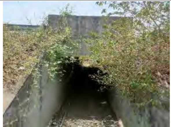
Box Culvert at Km 42+387
