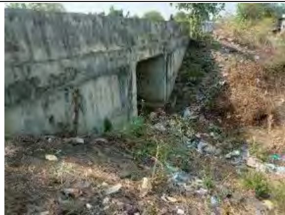
Box Culvert at Km 134+395
