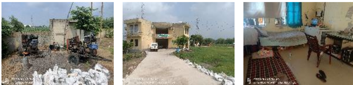
Figure 2-4. Facilities at Raibha Toll Plaza
