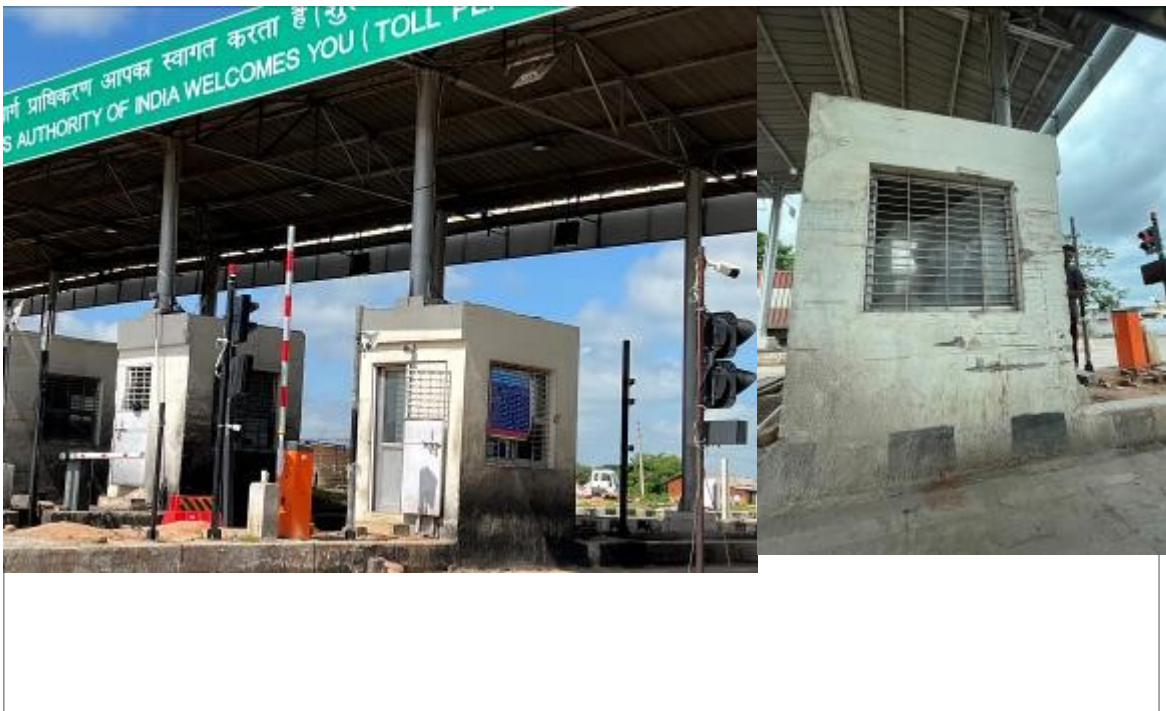
Photo 2: Electronic Toll Collection (ETC) lanes and toll booths at the toll plaza
