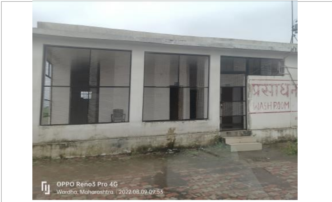
Photo 7: Washroom facility on the toll plaza
