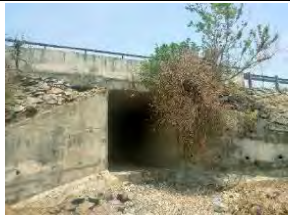
Box Culvert at Km 95+914
