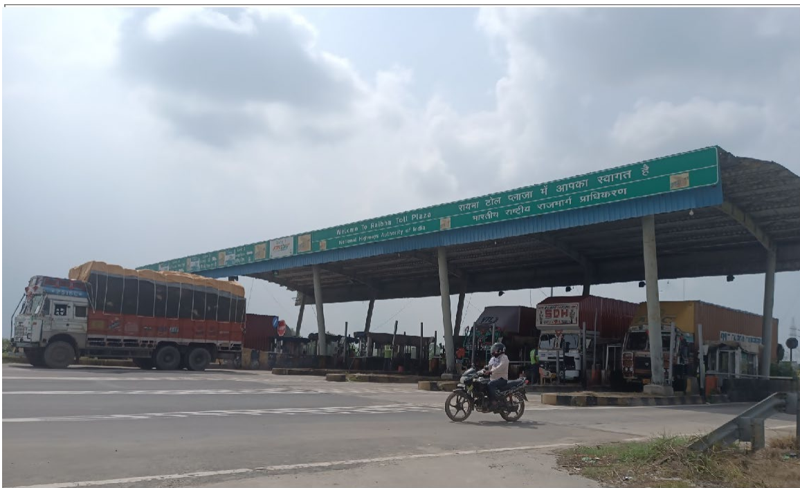
Photo 8: Raibha Toll plaza
