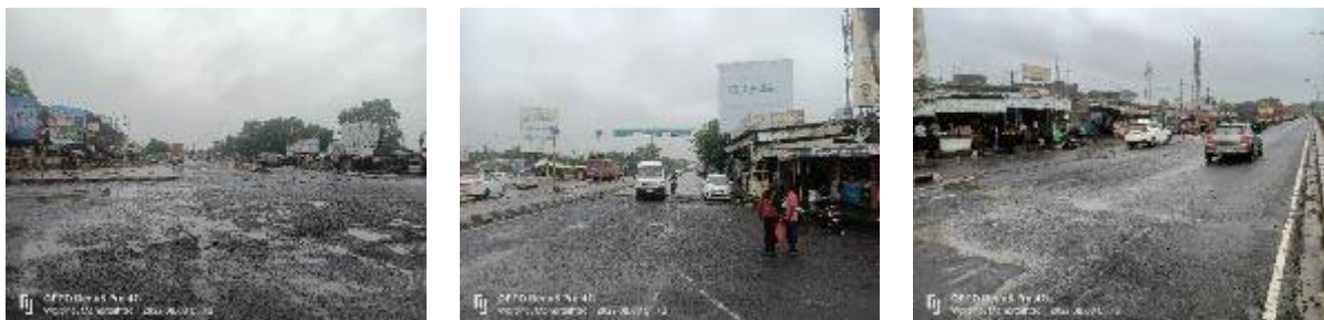
Figure 2-3. Encroachment Observed During the Site Visit on 9-10 August 2022
