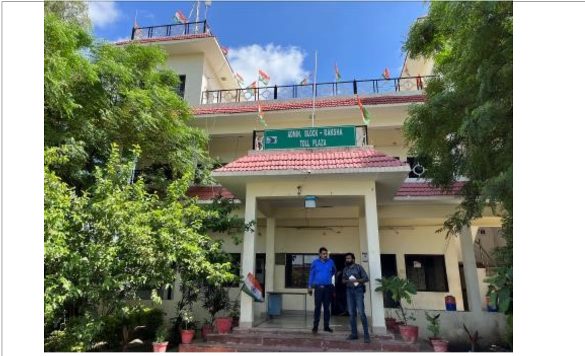
Photo 1: Toll plaza building
