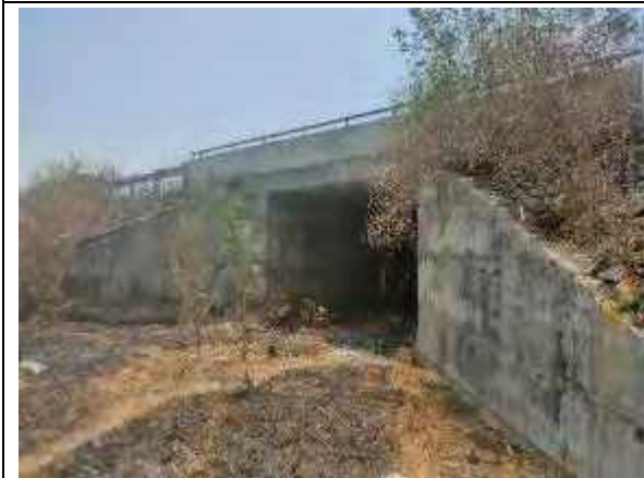
Box Culvert at Km 93+985
