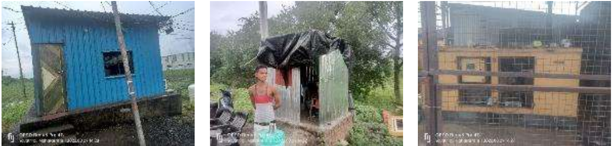
Figure 2-5. Kelapur Toll Plaza
