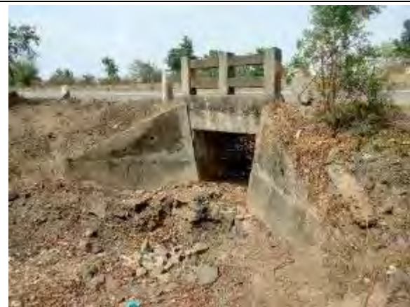
Slab Culvert at Km 57+155
