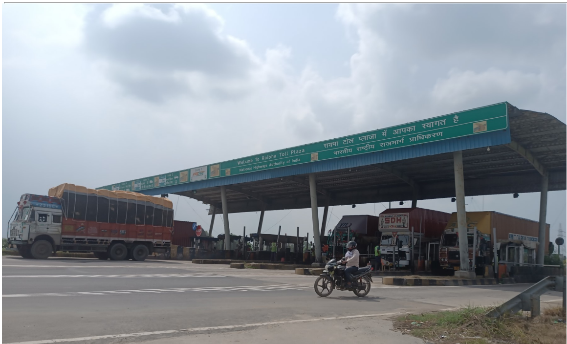
Photo 8: Raibha Toll plaza
