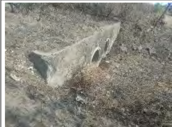
Pipe Culvert at Km 61+789
