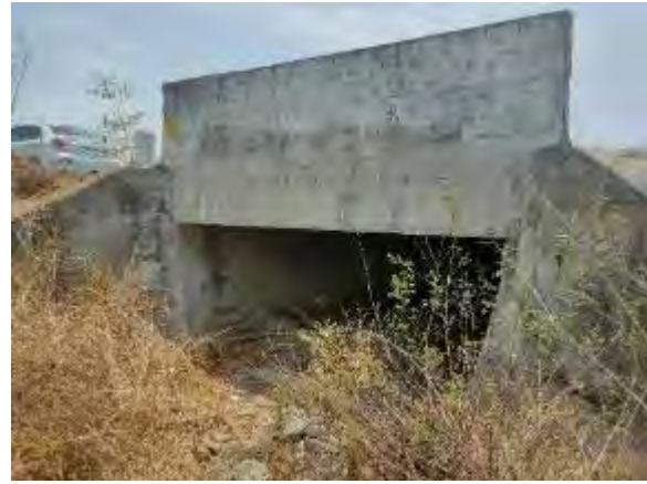
Slab Culvert at Km 45+985
