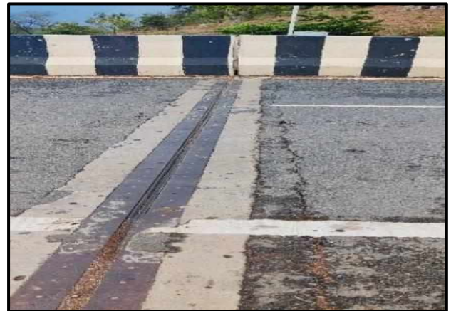
Major Bridge at Ch. 1319+870
