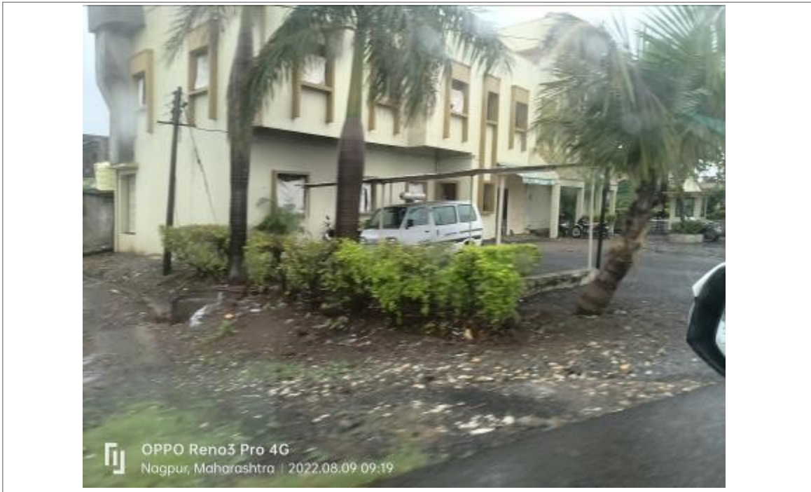
Photo 1: Toll plaza building
