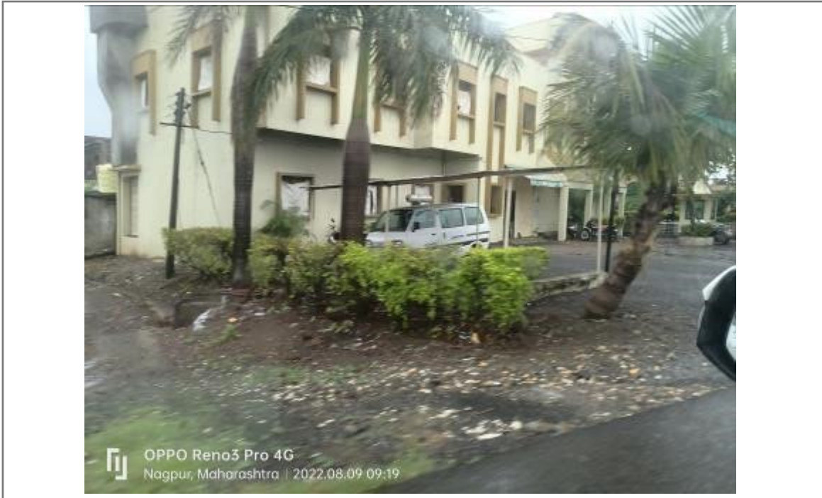
Photo 1: Toll plaza building
