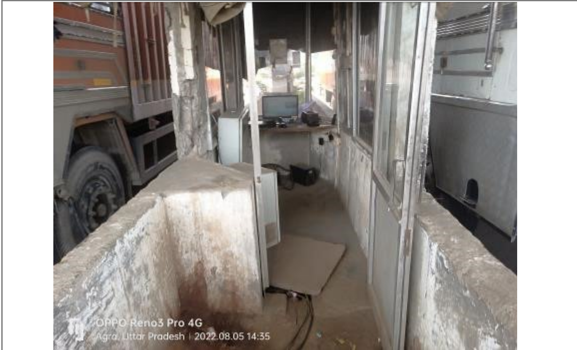
Photo 9: Inside view of toll booth
