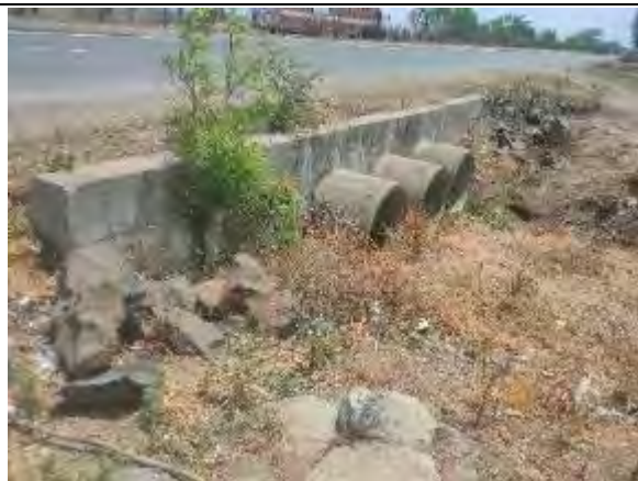
Pipe Culvert at Km 90+720
