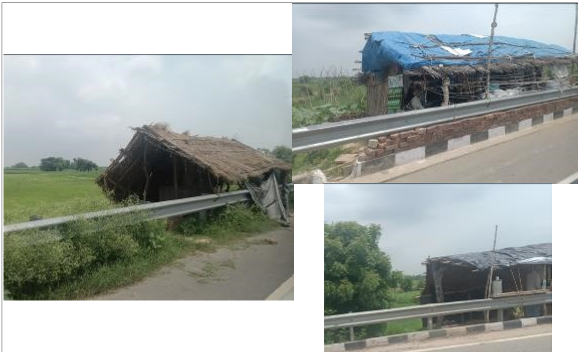
Photo 2: Encroachments in the ROW
