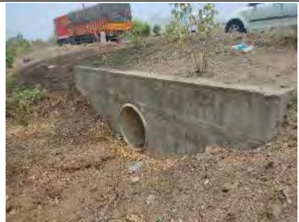
Pipe Culvert at Km 39+249
