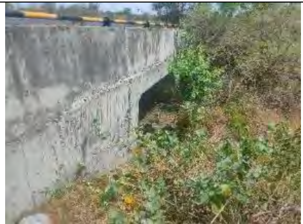
Box Culvert at Km 83+092
