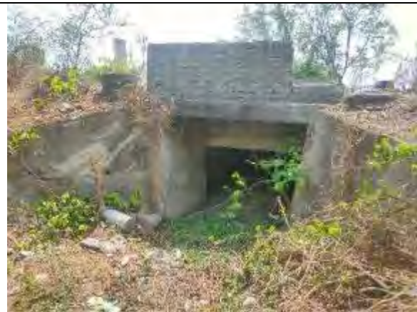
Slab Culvert at Km 51+180
