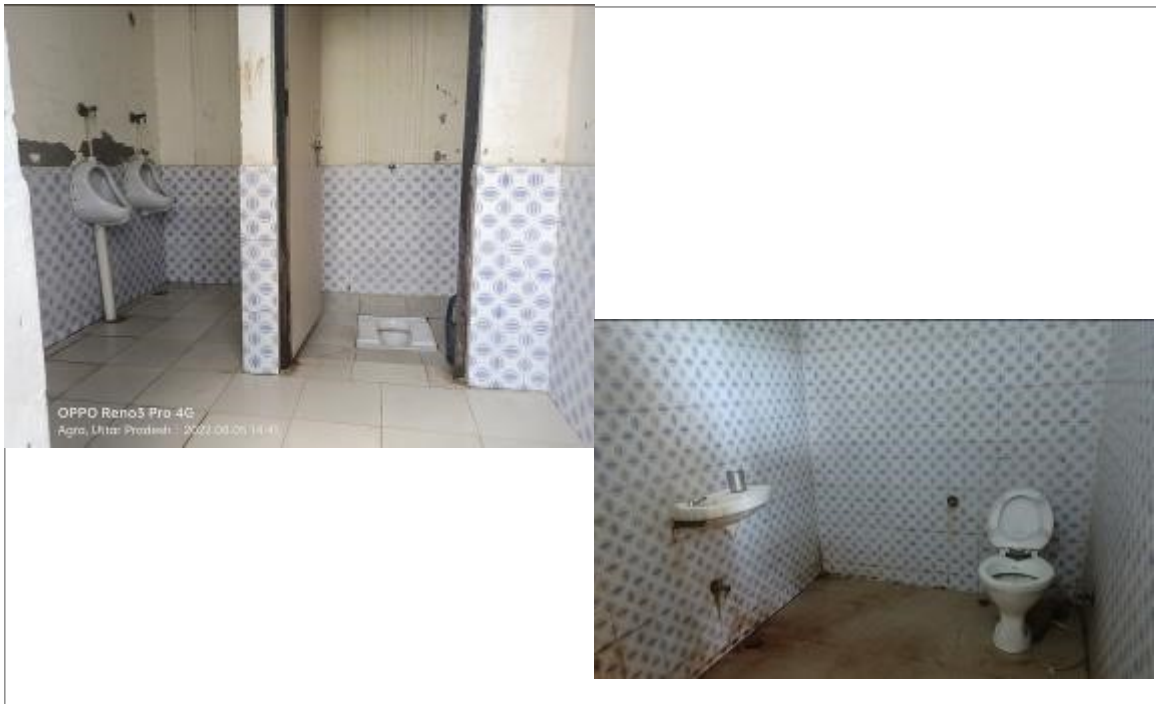
Photo 6: Toilet facilities at the toll plaza
