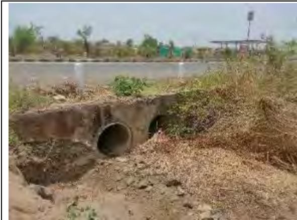
Pipe Culvert at Km 38+483
