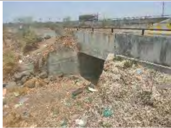
Box Culvert at Km 100+121
