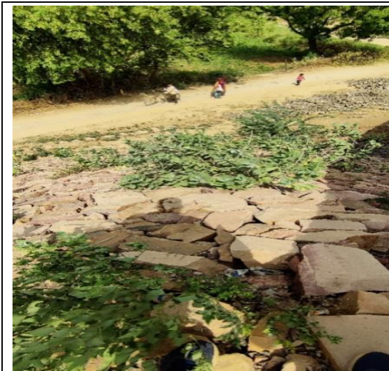
MNBR at CH. 17+661
