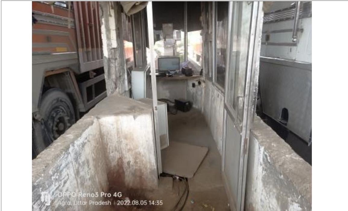
Photo 9: Inside view of toll booth
