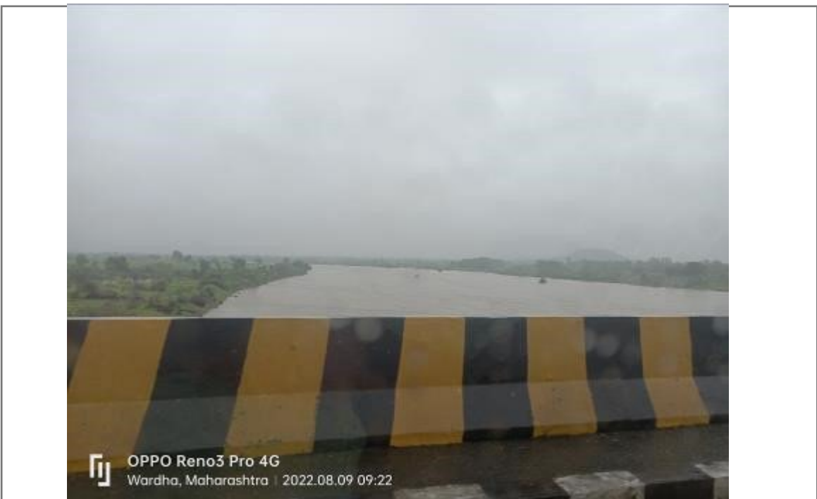
Photo 2: Bridge over the river in project area
