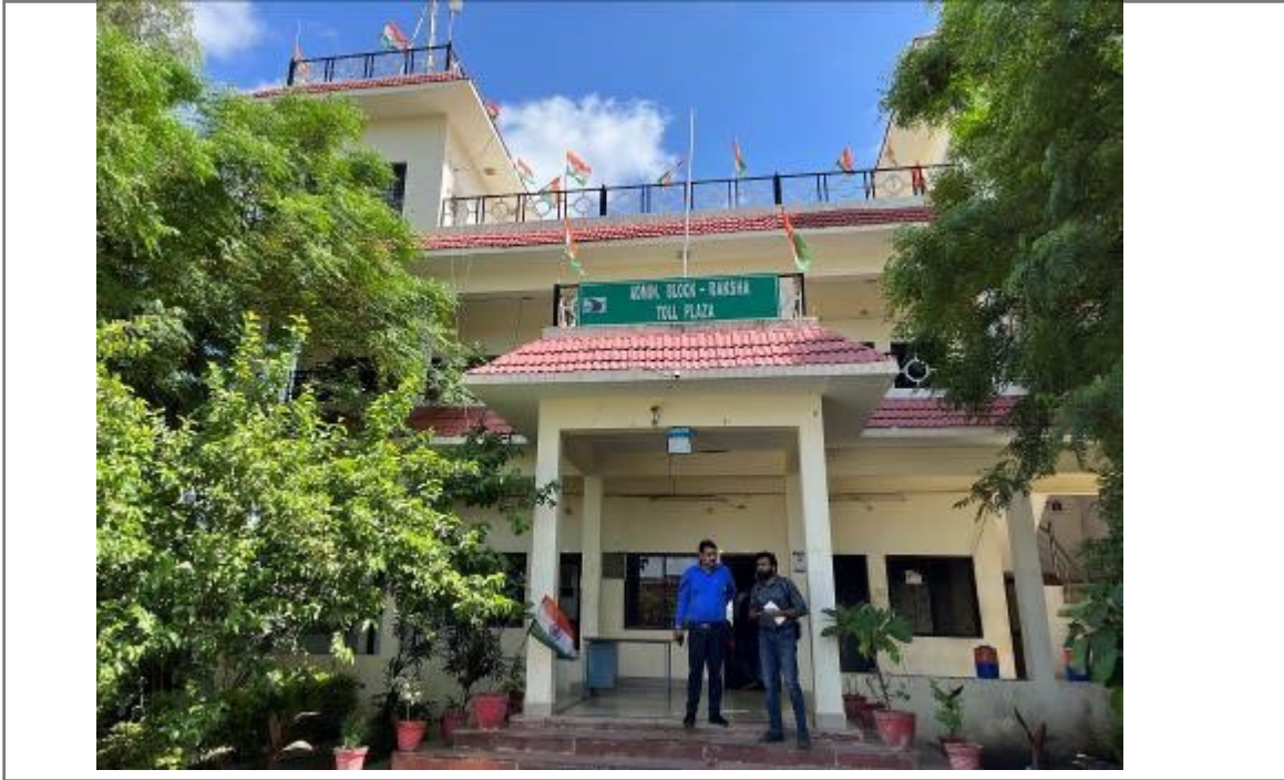
Photo 1: Toll plaza building
