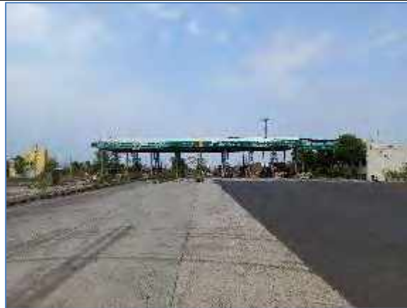
Toll Plaza at km 92+500
