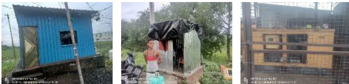
Figure 2-5. Kelapur Toll Plaza
