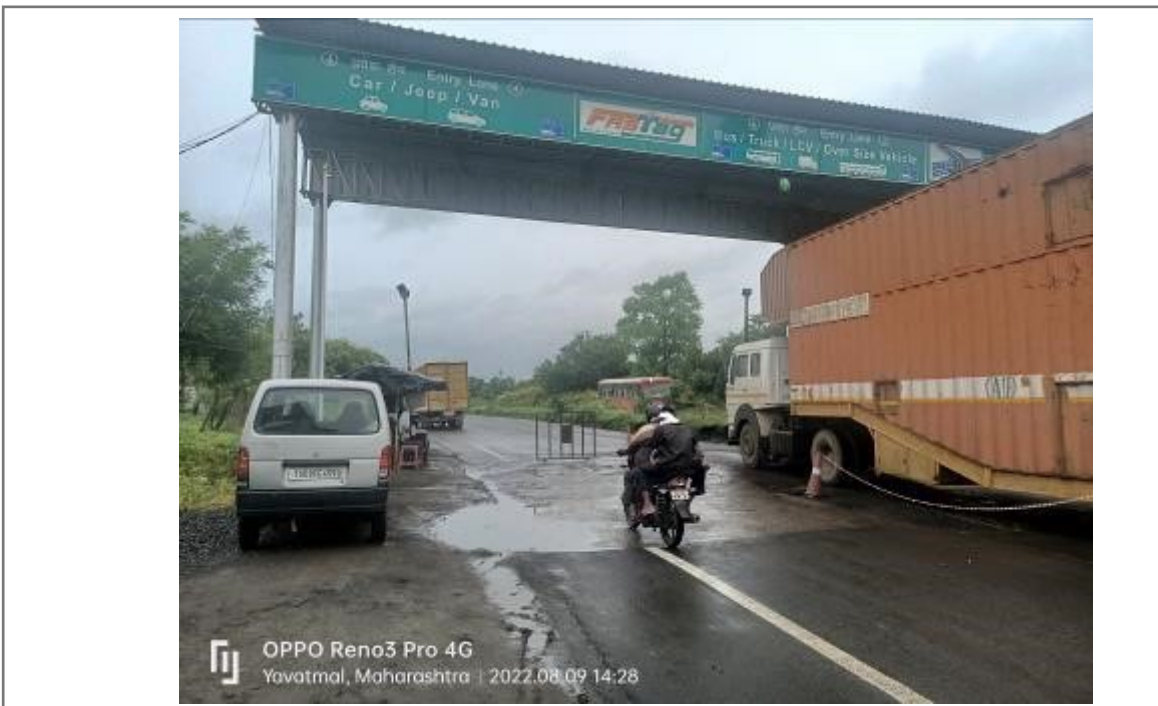
Photo 9: Electronic Toll Collection (ETC) lane
