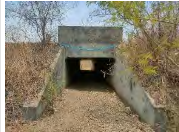
Box Culvert at Km 41+016
