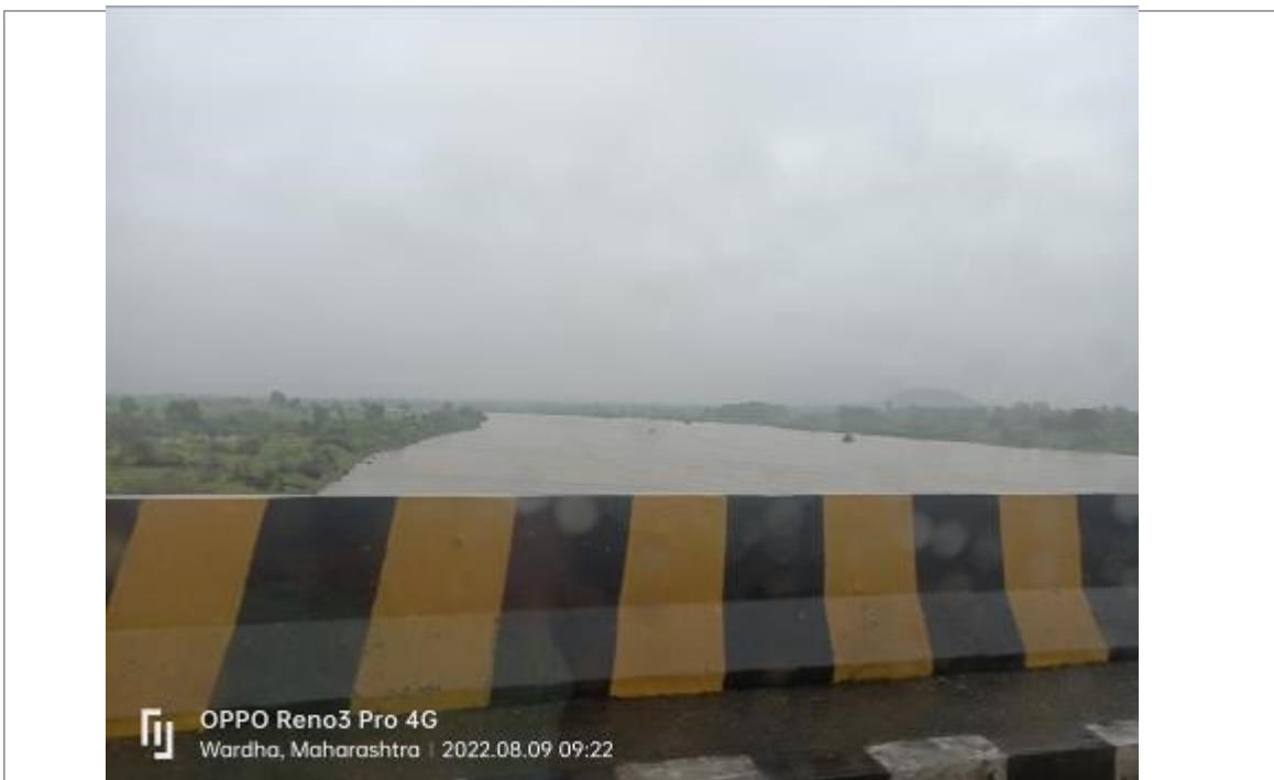
Photo 2: Bridge over the river in project area
