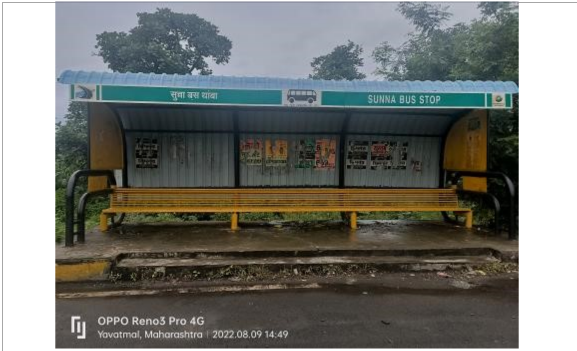
Photo 10: Bus stop along National highway
