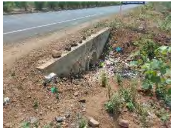
Pipe Culvert at Km 168+421
