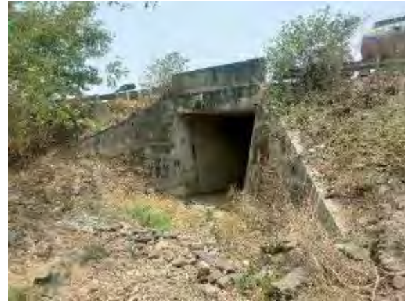
Slab Culvert at Km 42+335
