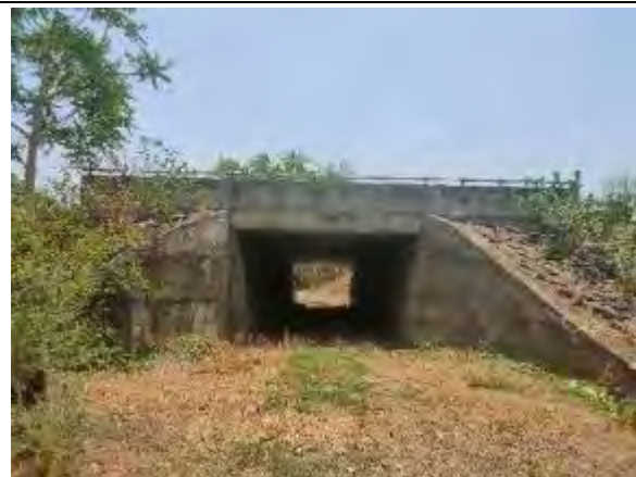
Slab Culvert at Km 164+145
