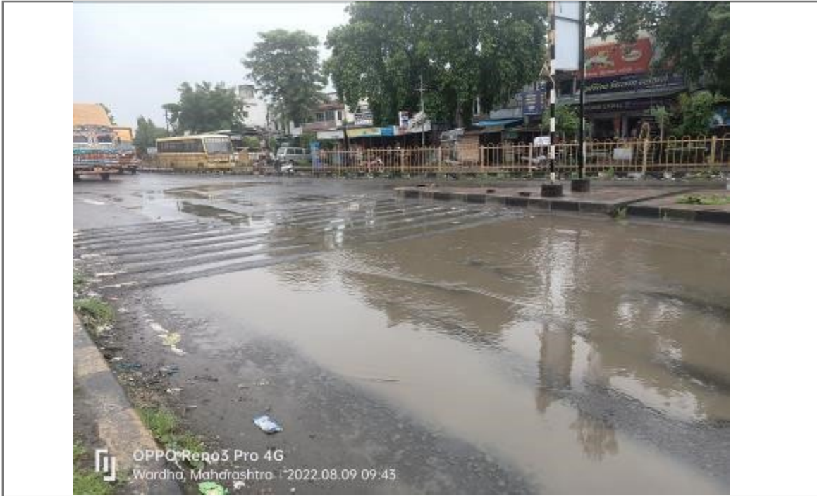
Photo 3: Water logging on the road in project area
