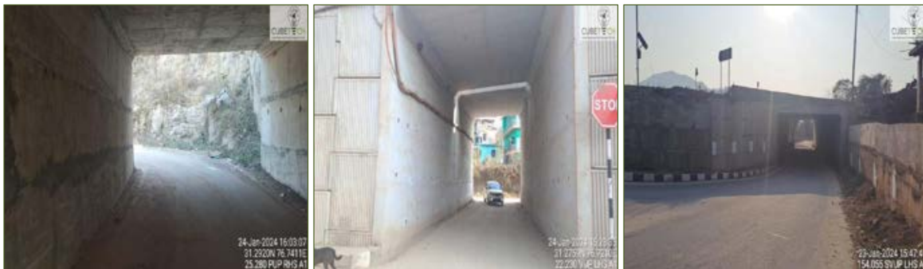
Figure 4-6: Condition of Underpasses
