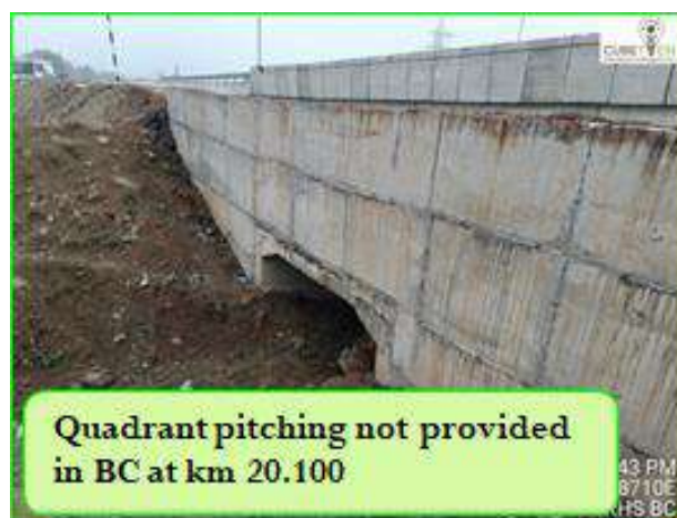
Figure 4-8: Condition of Culverts
