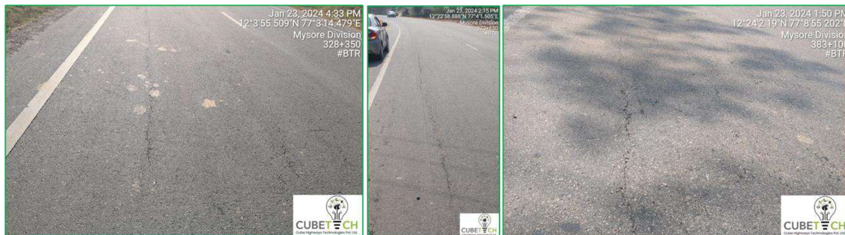
Figure 7-6: Longitudinal Cracks
