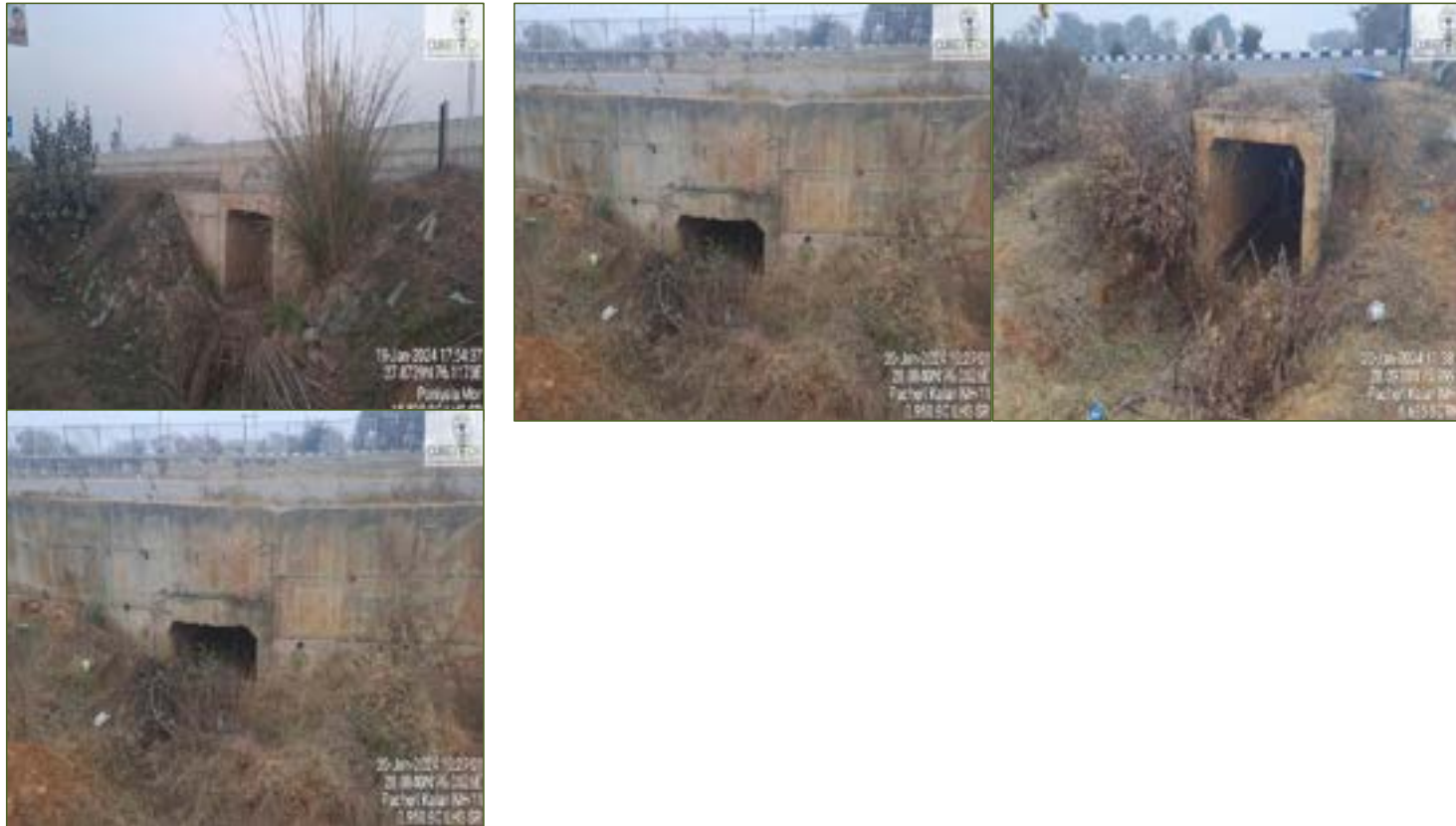
Figure 4-5: Condition of Culvert
