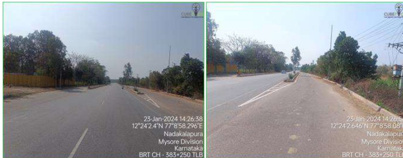
Figure 3-8: Truck Lay bye
