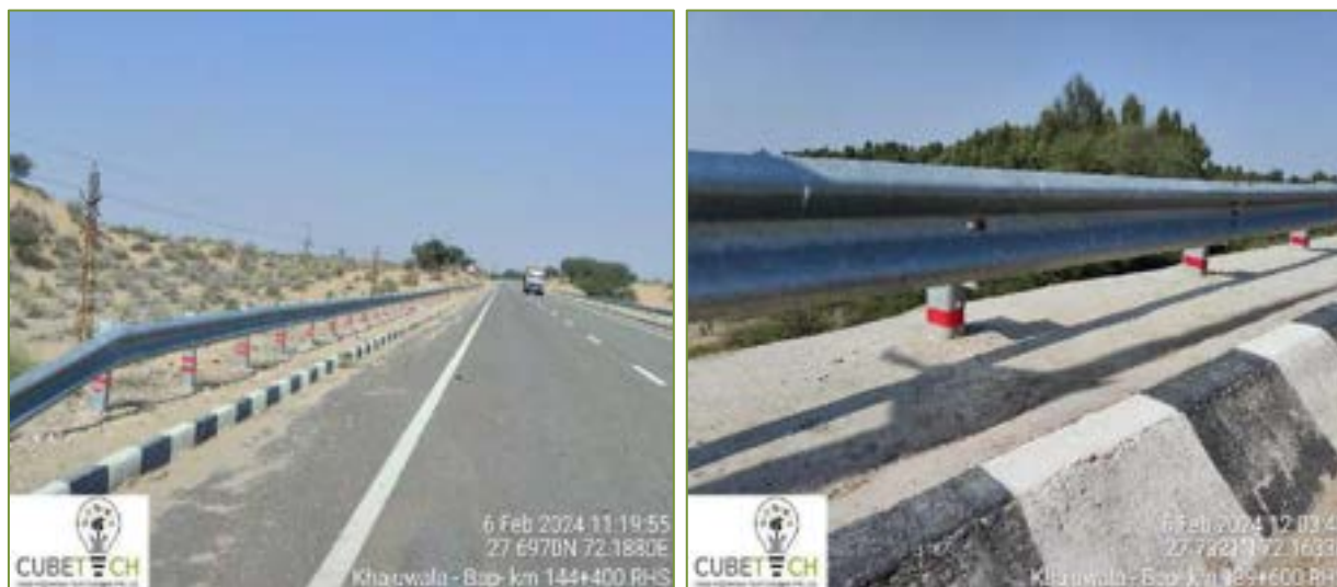
Figure 3-5: Metal beam crash barrier (MBCB) along the project stretch
