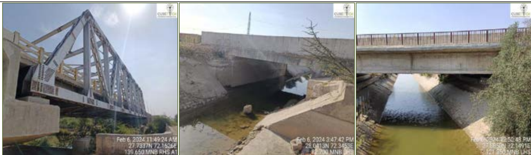
Figure 4-1: Condition of Minor Bridges
