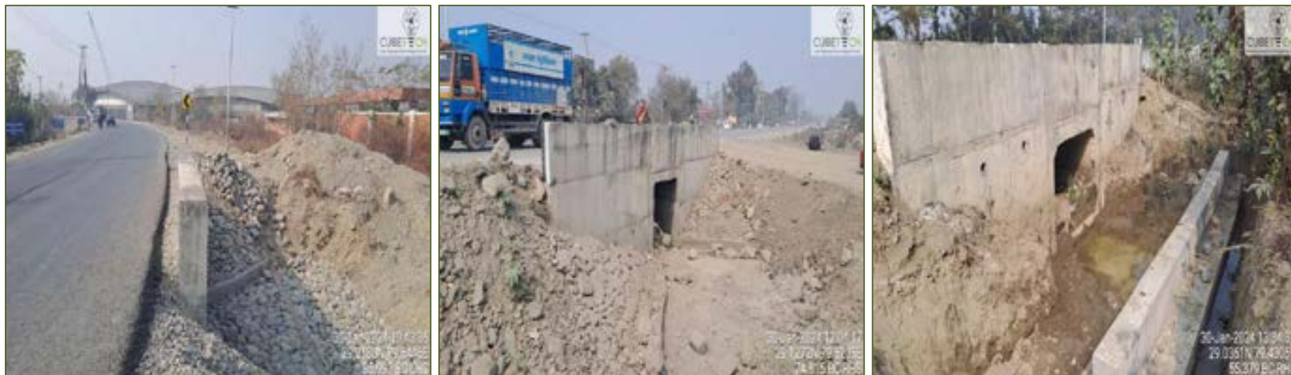
Figure 4-6: Condition of Culverts
