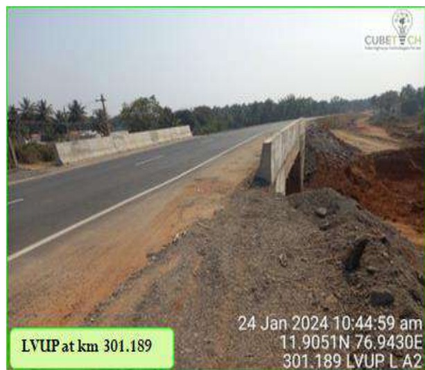
Figure 4-5: Condition of LVUP's
