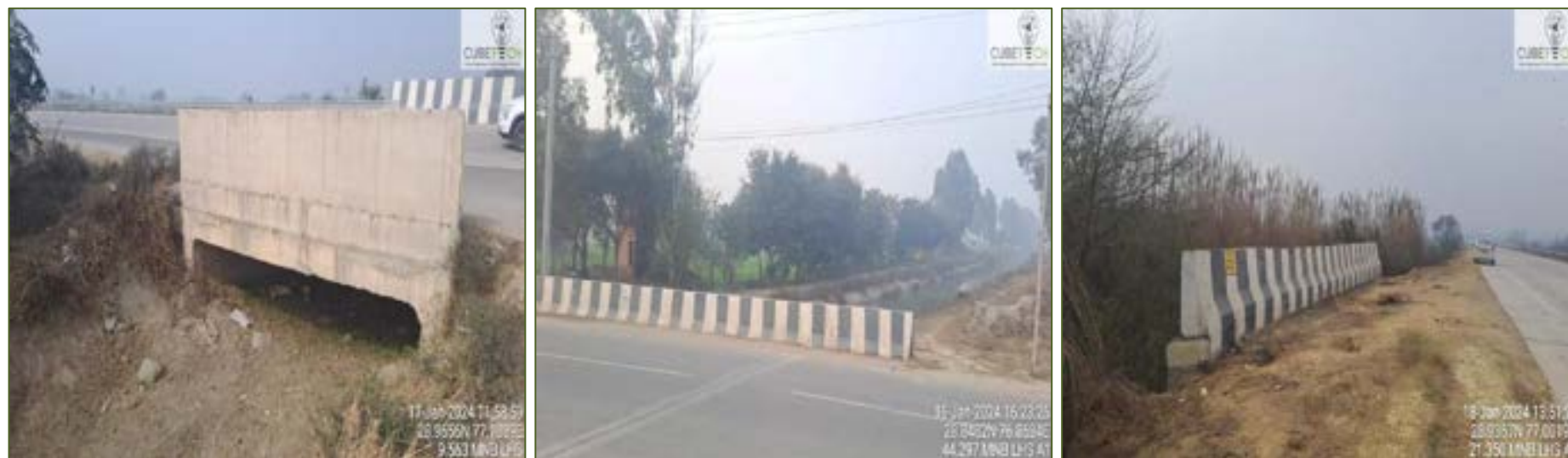
Figure 4-1: Condition of Minor Bridges
