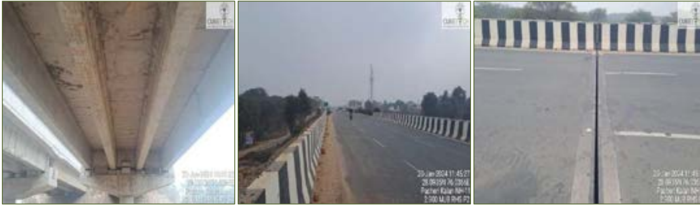
Figure 4-1: Condition of Major Bridges
