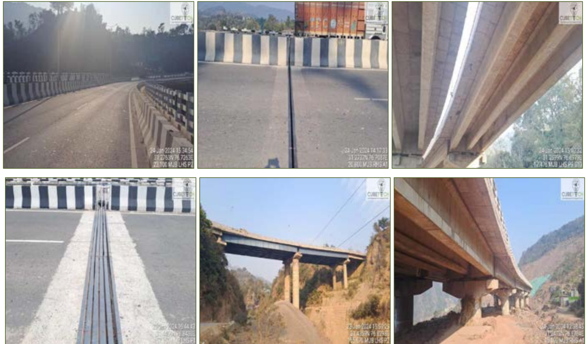
Figure 4-1: Condition of Major Bridge
