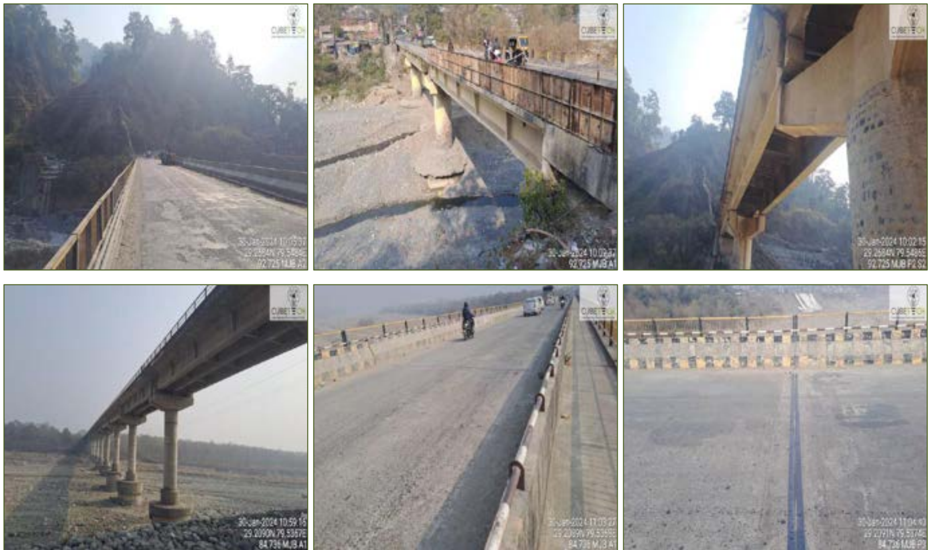
Figure 4-1: Condition of Major Bridges
