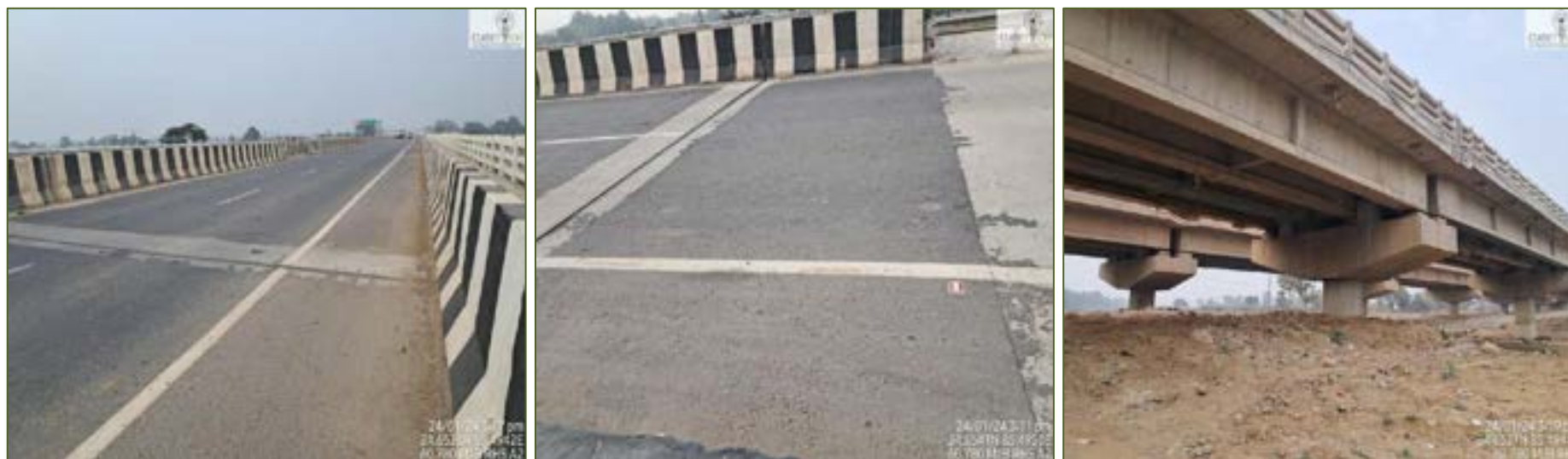
Figure 4-1: Condition of Major Bridges
