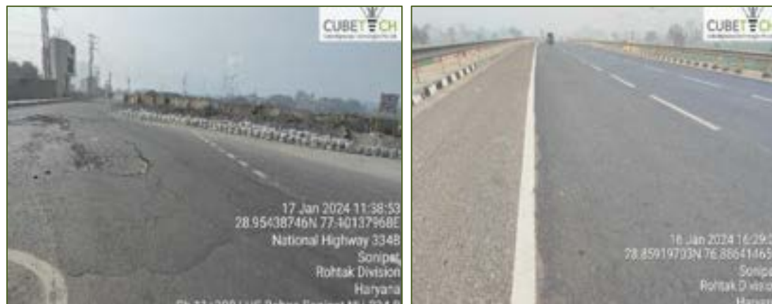
Figure: Alligator Cracks
