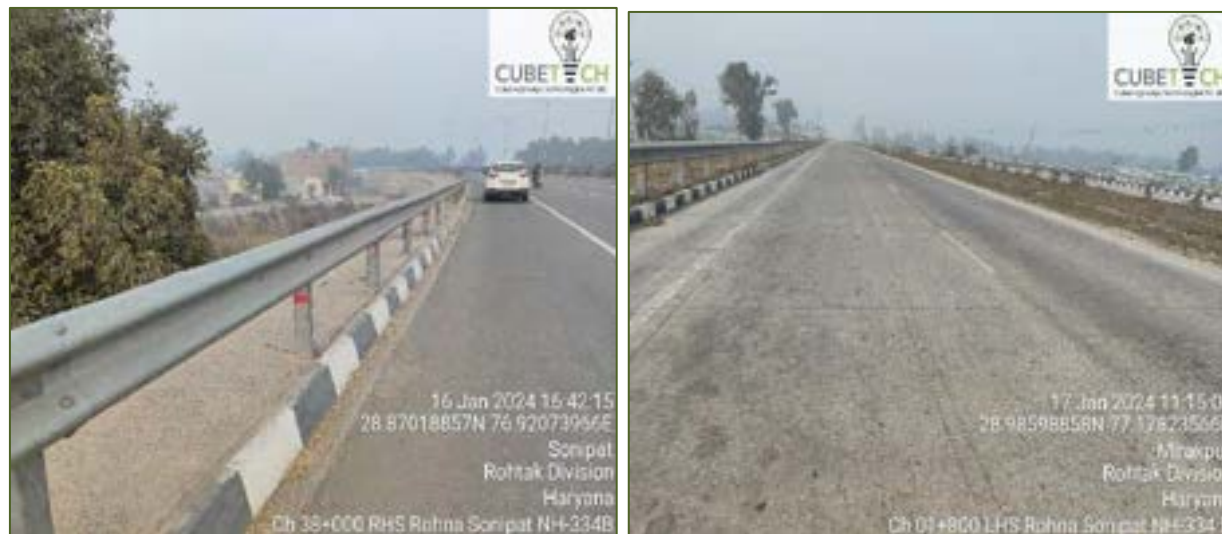
Figure 3-4: Safety crash barrier (MBCB) along the project stretch
