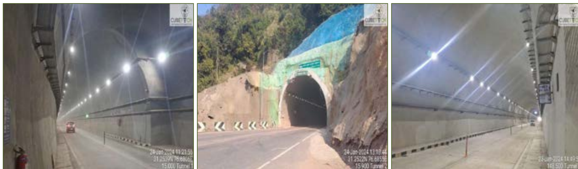
Figure 4-5: Condition of Tunnels
