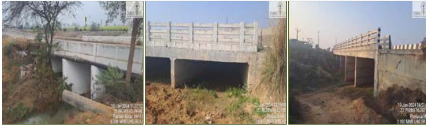
Figure 4-2: Condition of Minor Bridges
