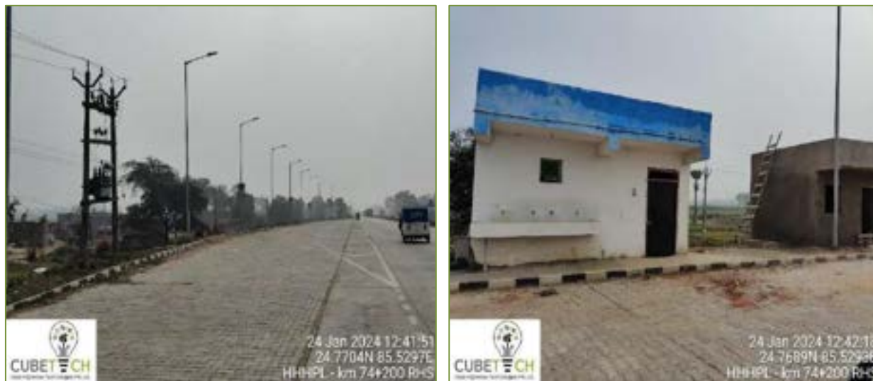
Figure 3-10: Truck Lay bye
