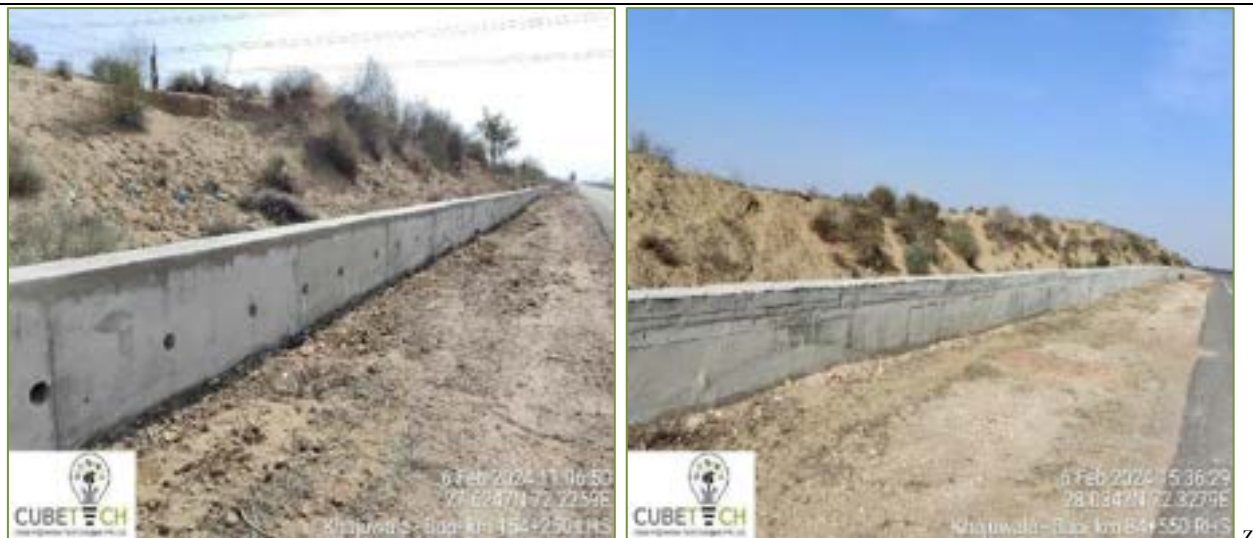
Figure 3-8: Retaining wall
