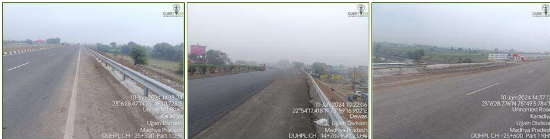
Figure 3-5: Safety crash barrier (MBCB) along the project stretch
