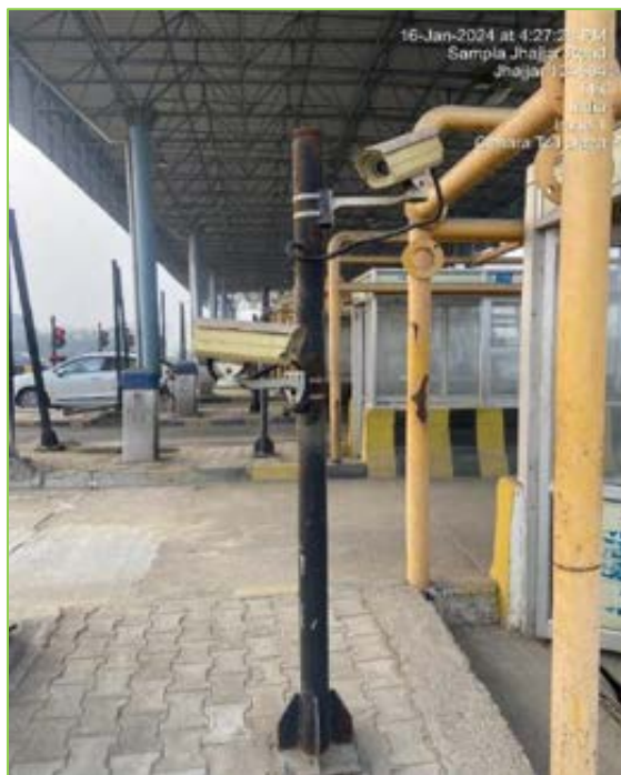
Figure 3-15: LPIC and ICS Cameras.
