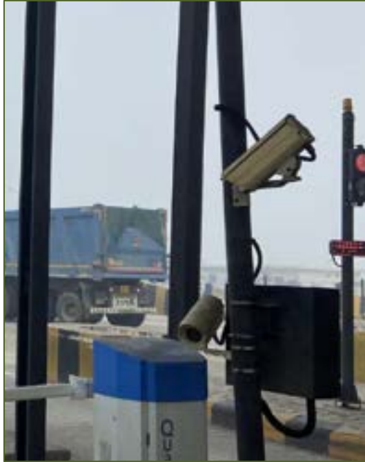
Figure 3-14: LPIC and ICS Cameras.
