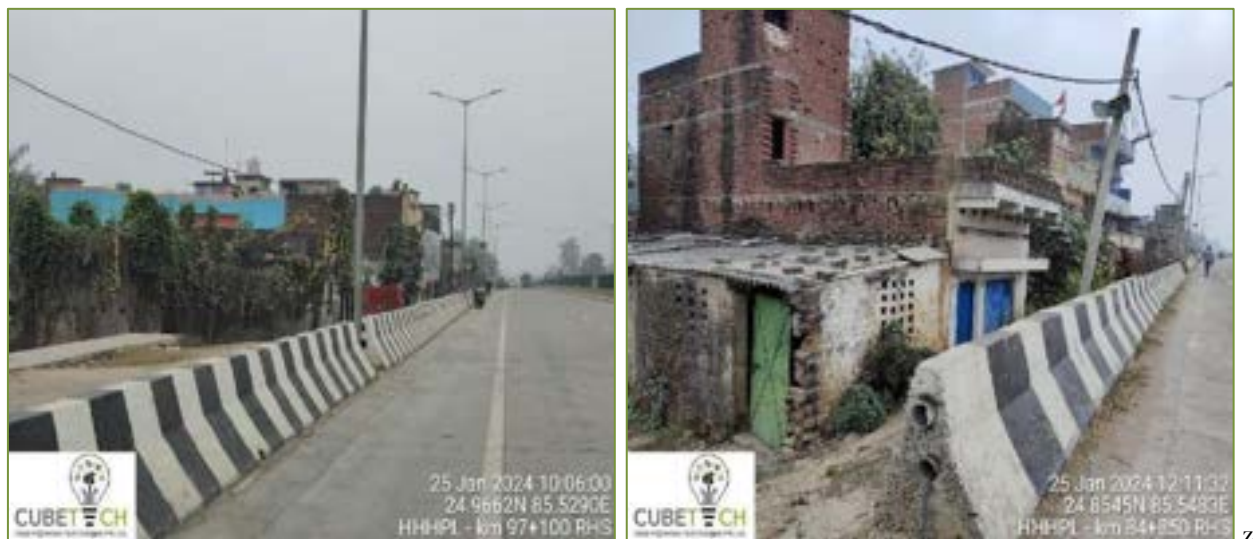
Figure 3-7: Rigid Crash Barrier
