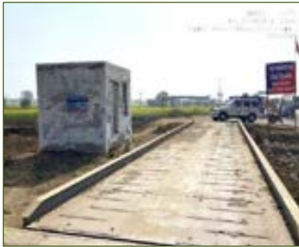
Figure 3-16: Static Weigh Bridge (SWB).
