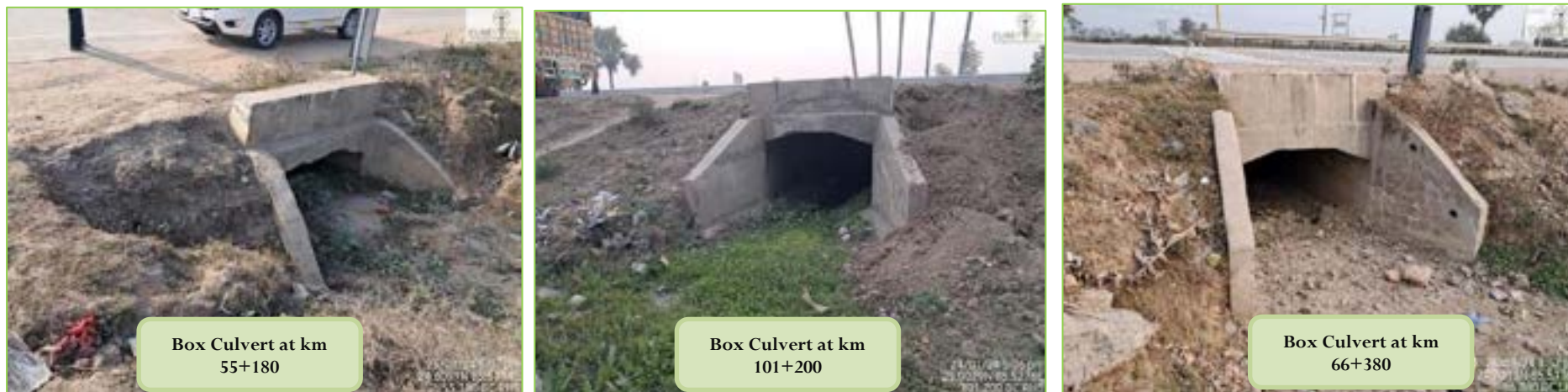
Figure 4-7: Condition of Box Culverts
