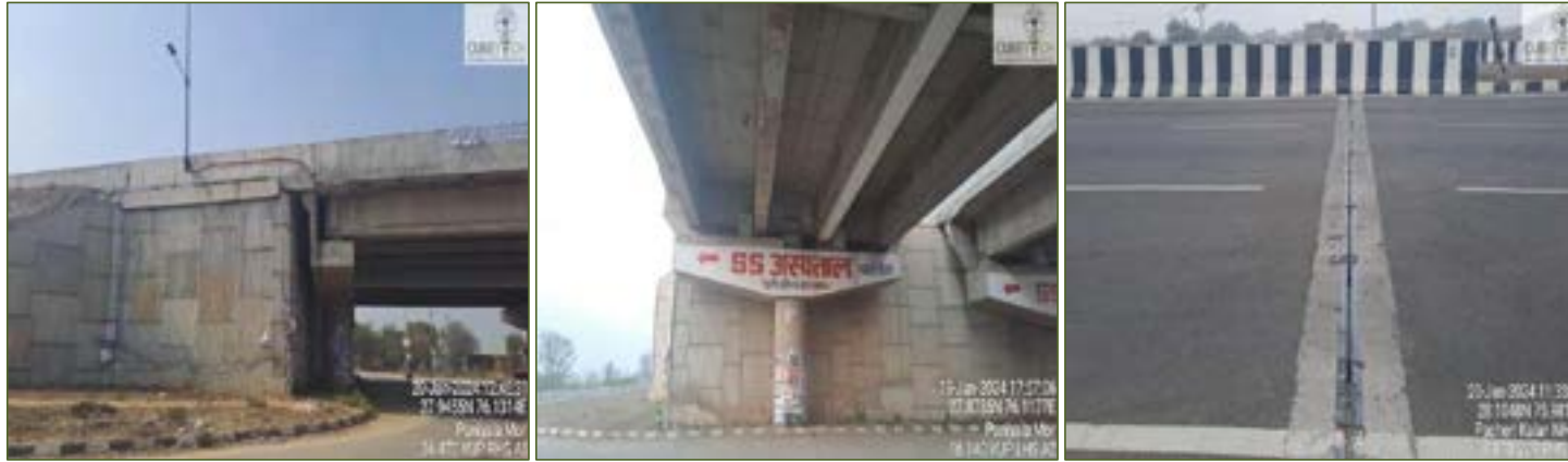
Figure 4-3: Condition of Vehicular Underpasses
