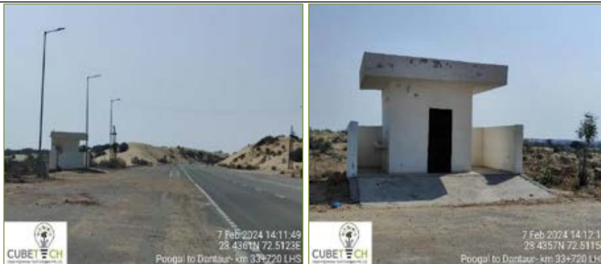
Figure 3-11: Truck Lay bye
