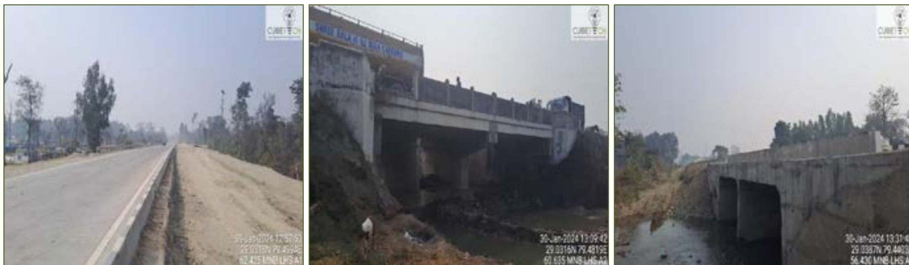
Figure 4-2: Condition of Minor Bridges
