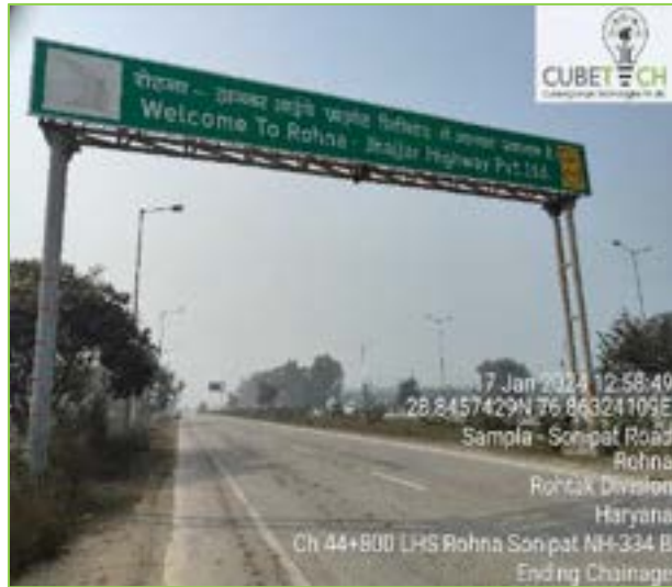
Figure 3-5: Overhead & Cantilever Gantry boards Highway Lighting
