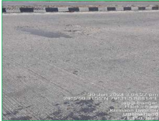
Figure: Scaling
