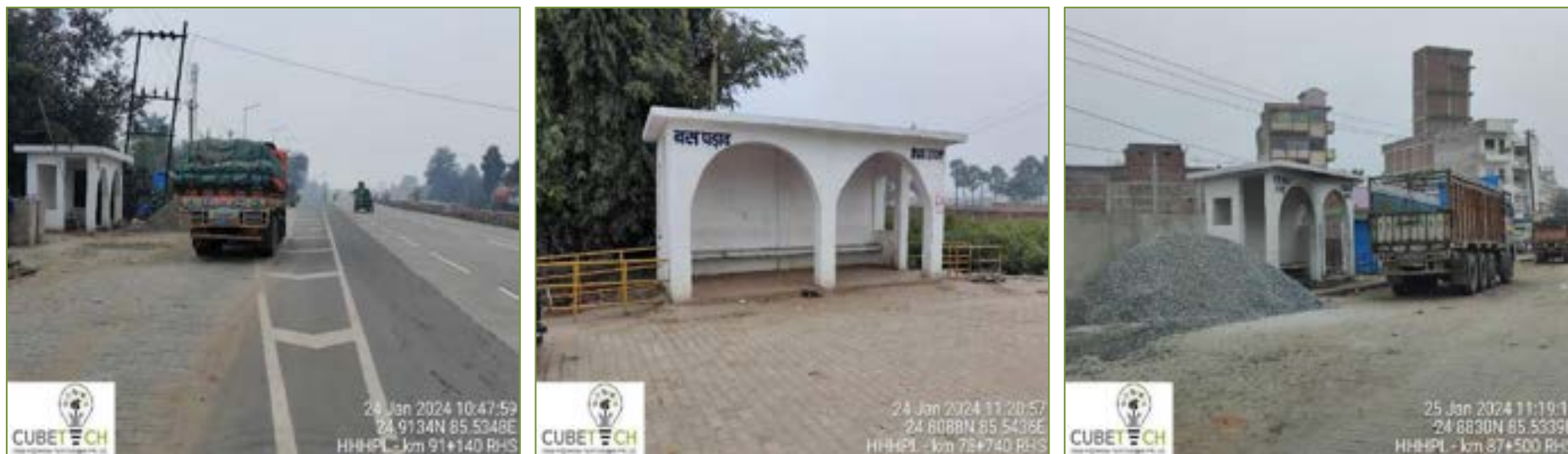
Figure 3-9: Bus bays / shelters
