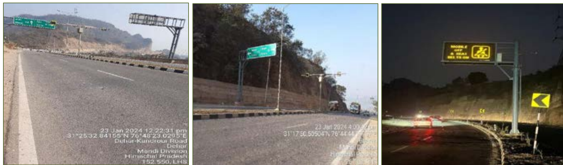
Figure 3-5: Overhead & Cantilever Gantry boards and VMS
