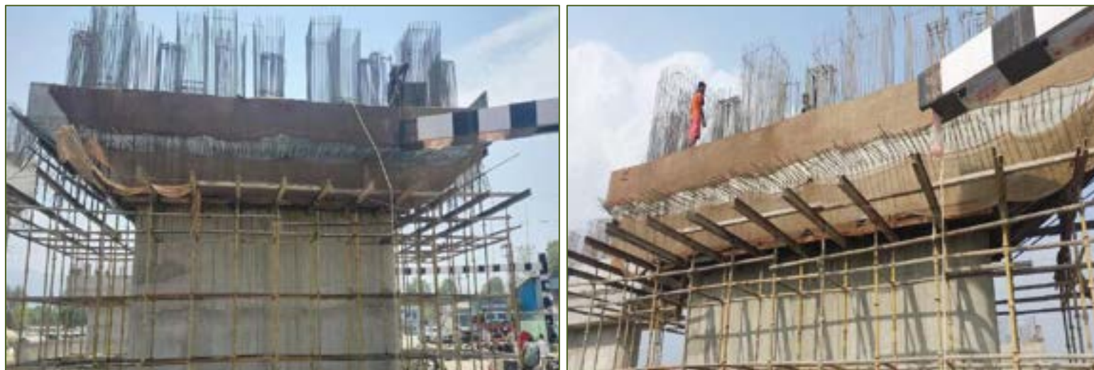
Figure 4-3: Progress of ROB
