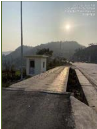
Figure 3-18: Static Weigh Bridge (SWB).
