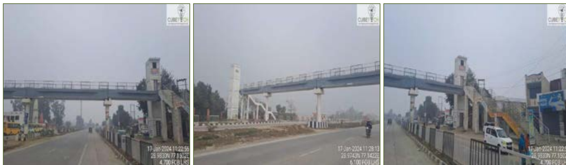
Figure 4-4: Foot Over Bridge at km 4.700 and km 5.980
