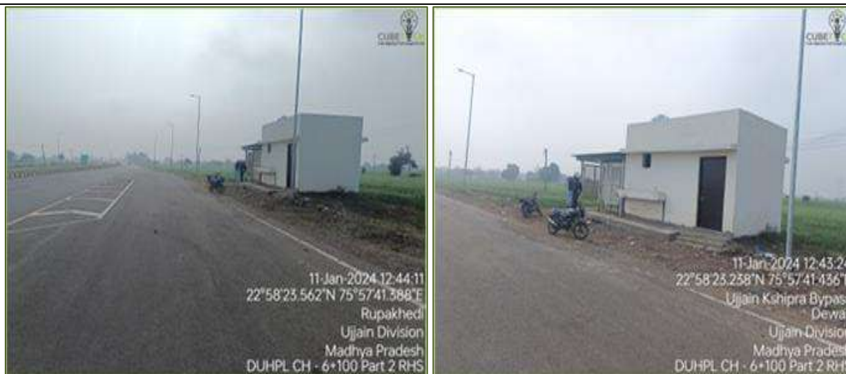
Figure 3-11: Truck Lay bye
