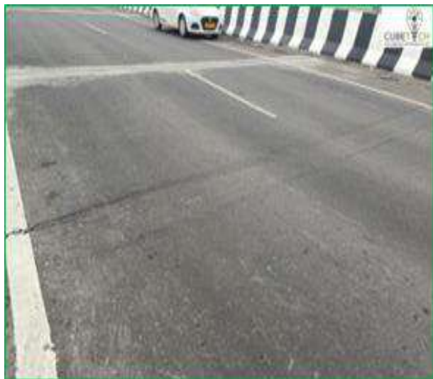
Figure 7-6: Transverse cracks
