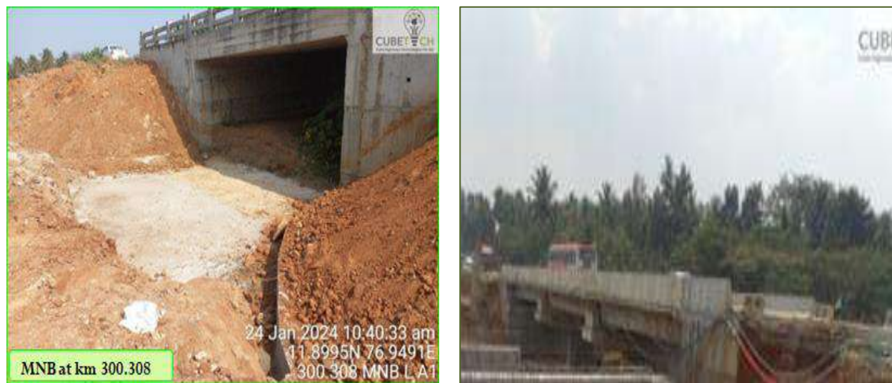
Figure 4-2: Condition of Minor Bridges at km 300+308 & 443+075
