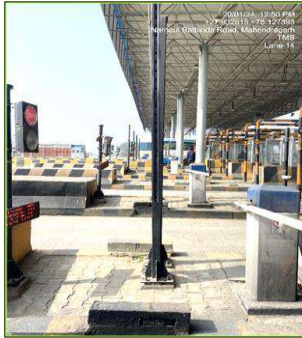
Figure 3-10: AVC Height Sensors
