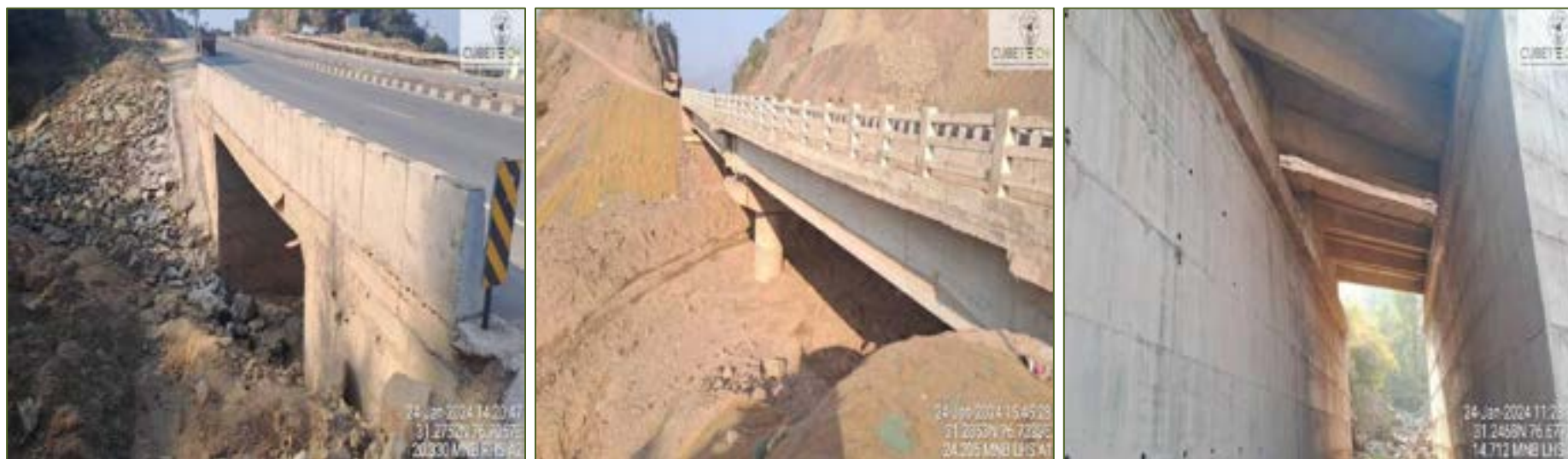
Figure 4-2: Condition of Minor Bridge
