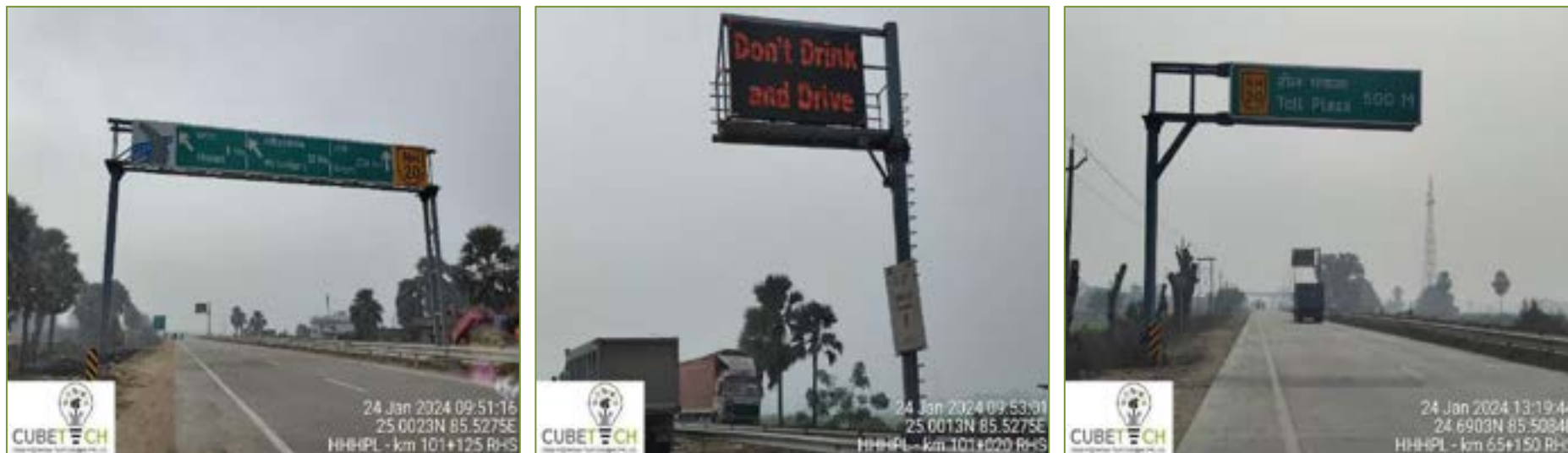
Figure 3-6: Overhead & Cantilever Gantry boards and VMS
