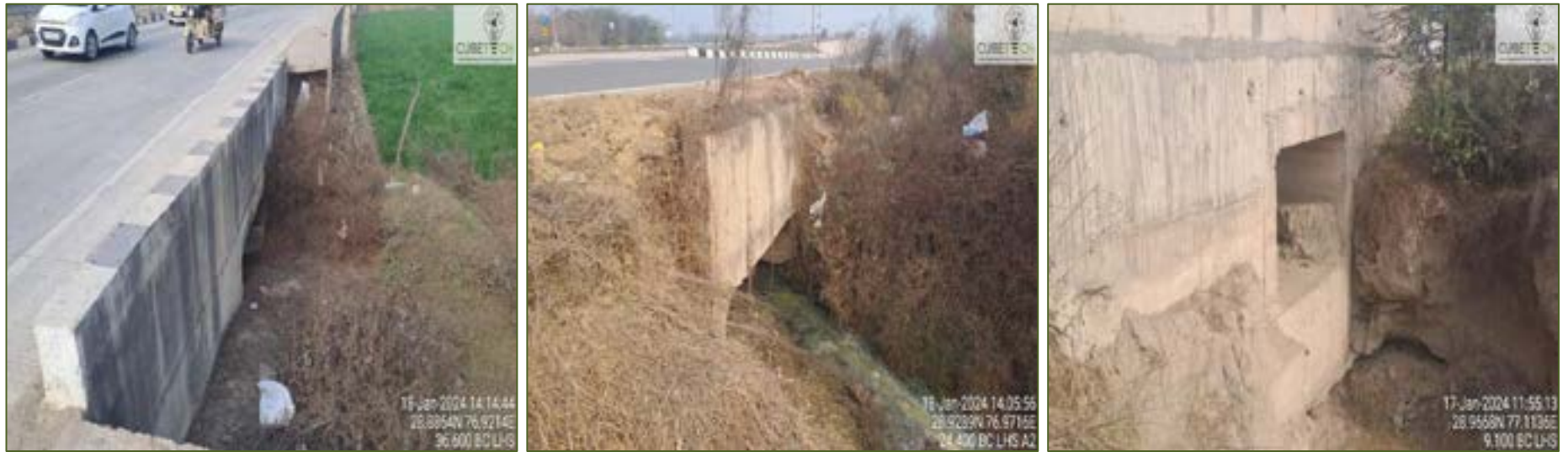
Figure 4-7: Condition of Culverts
