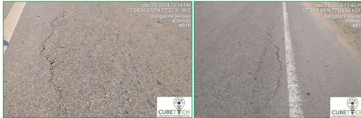
Figure 7-7: Alligator Cracks
