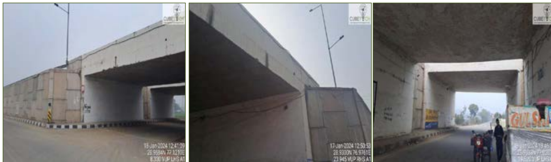
Figure 4-5: Condition of Vehicular Underpasses
