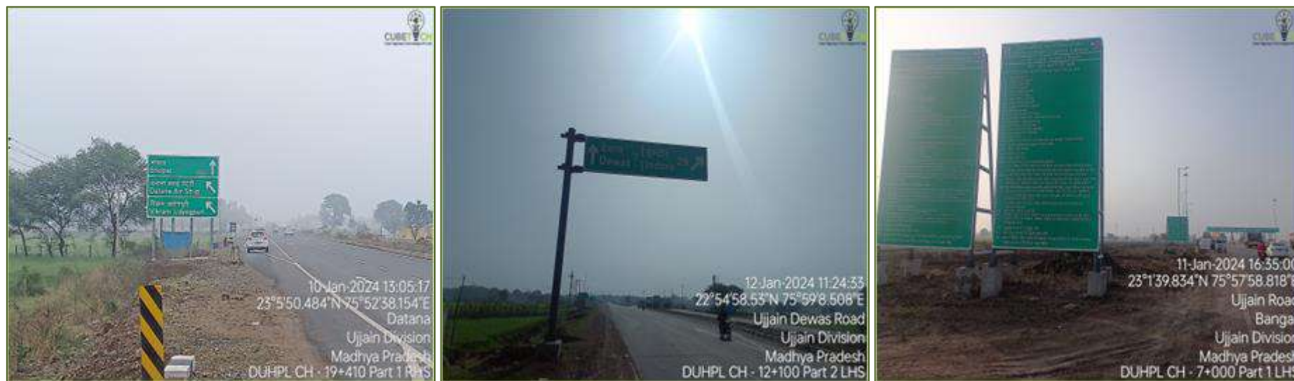
Figure 3-8: Traffic sign boards
