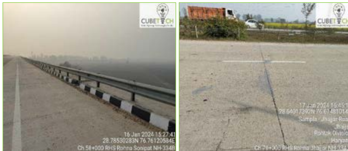
Figure 3-4: Crash barrier along the project stretch
