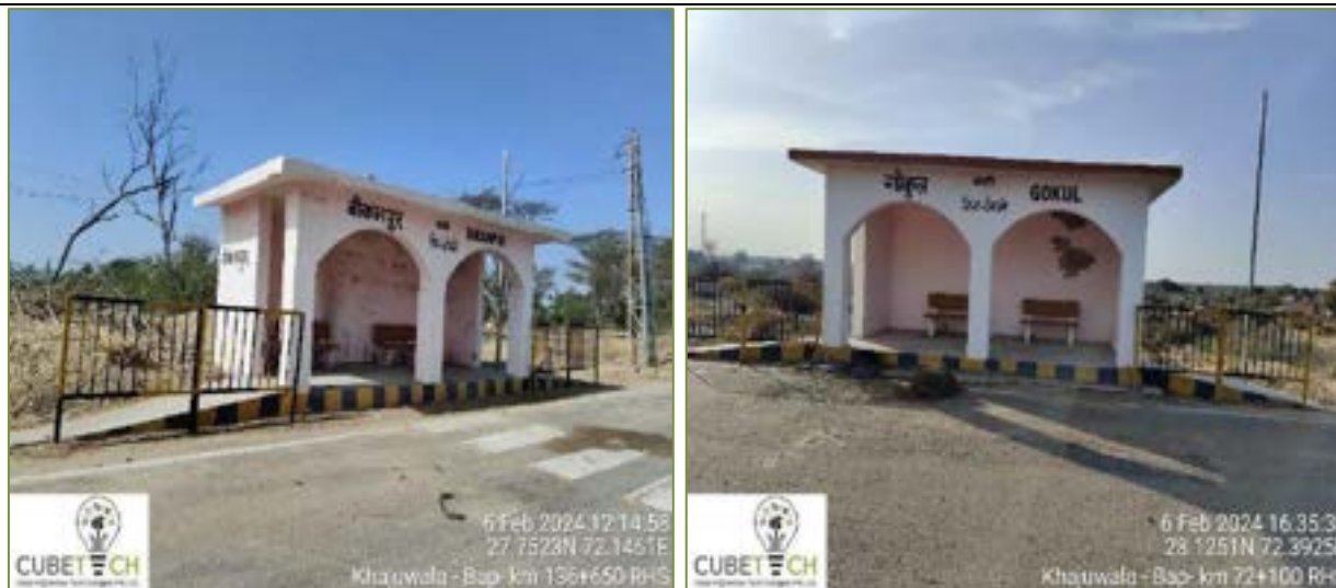
Figure 3-10: Bus bays / shelters
