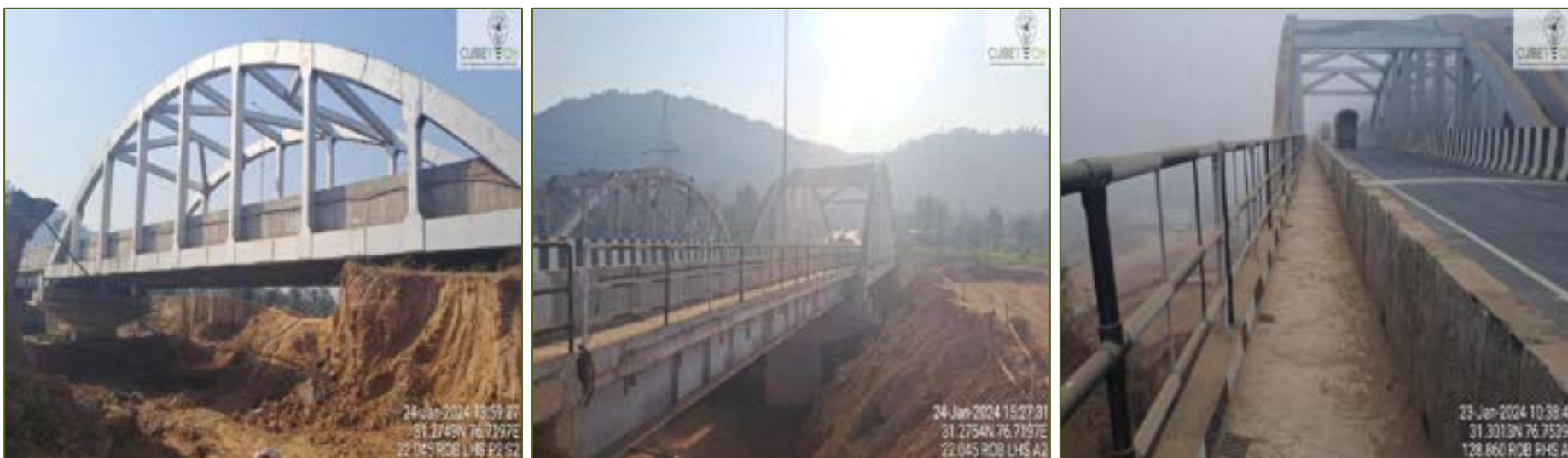
Figure 4-3: Condition of Road Over Bridges
