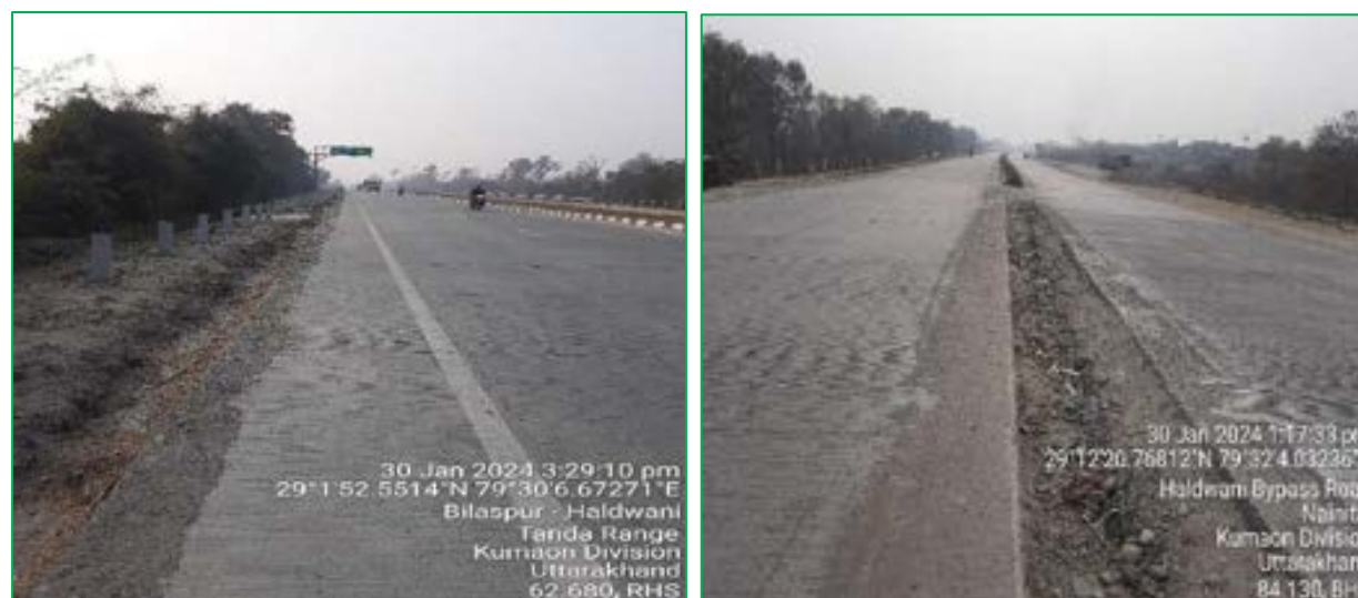
Figure 3-3: Safety crash barrier (MBCB) along the Project Stretch
