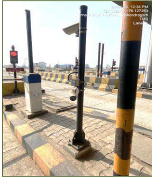
Figure 3-13: LPIC and ICS Cameras.
