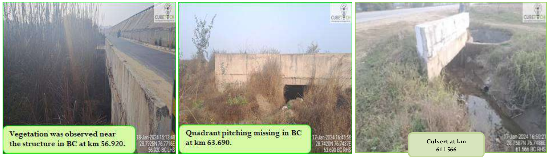
Figure 4-6: Condition of Culverts
