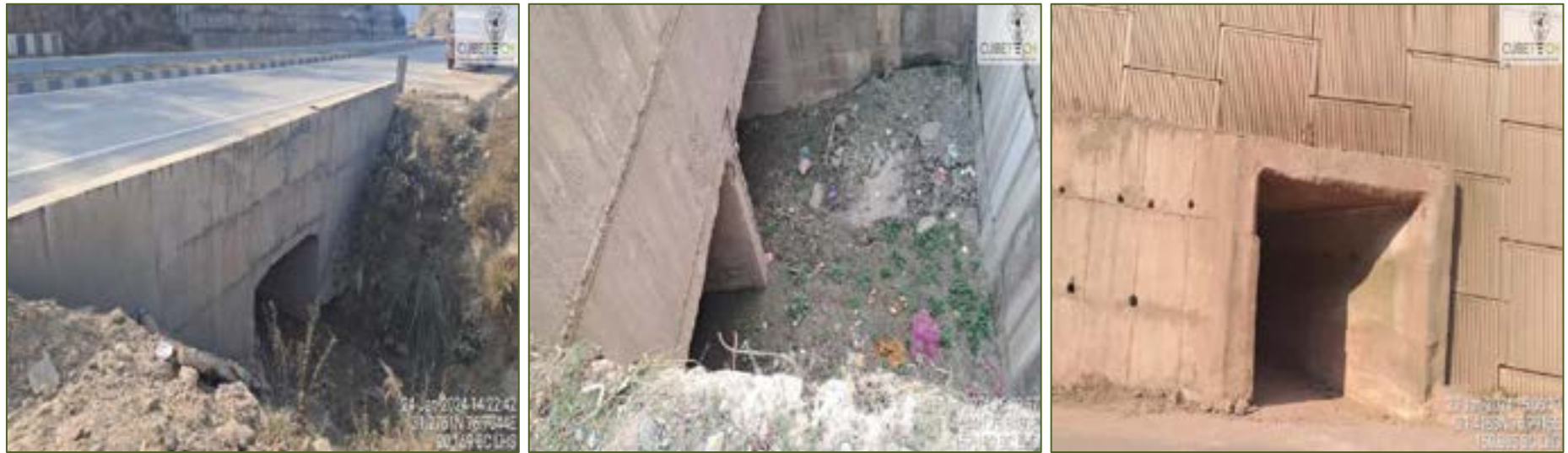
Figure 4-7: Condition of Culverts
