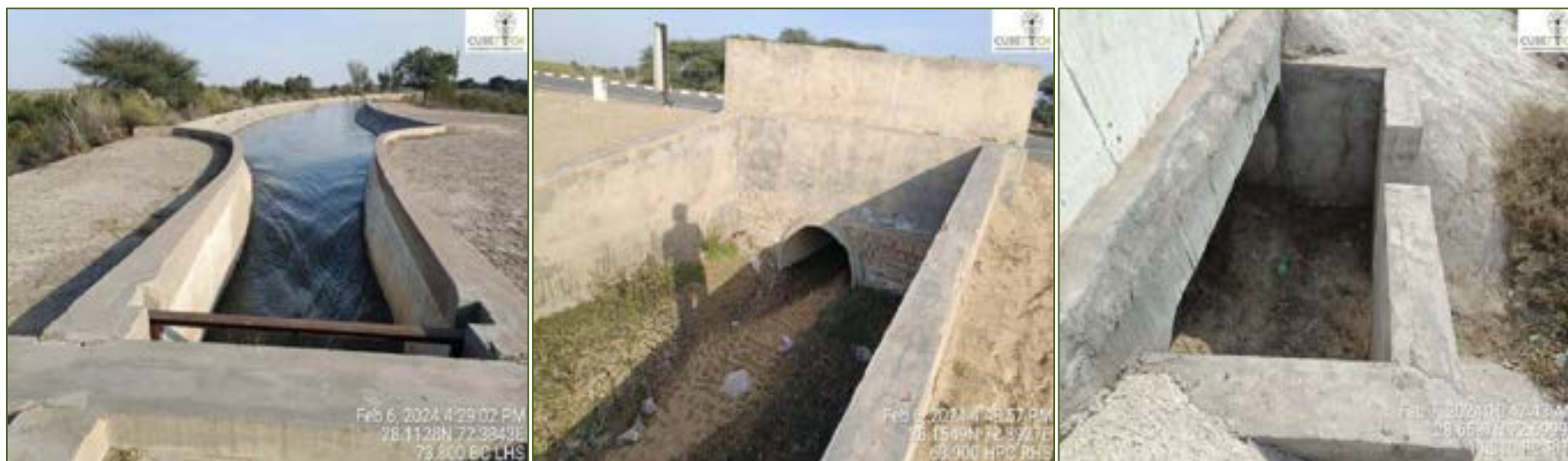
Figure 4-3: Condition of Box Culverts
