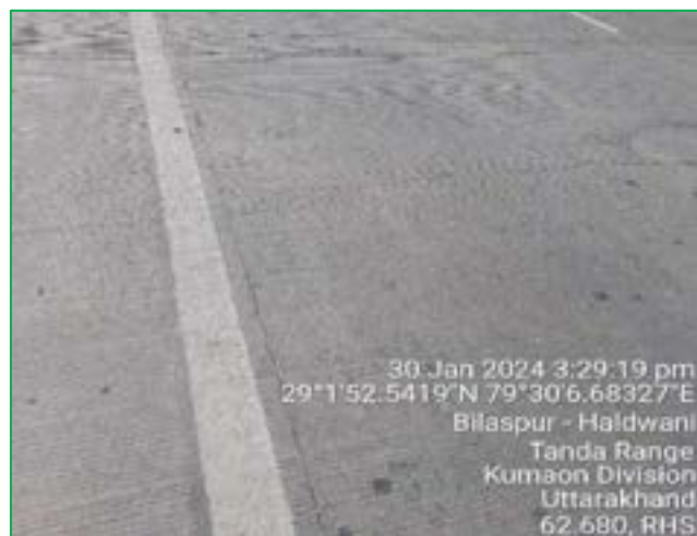
Figure 0-2: Transverse Cracks
