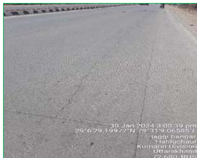
Figure 0-1: Longitudinal Cracks
