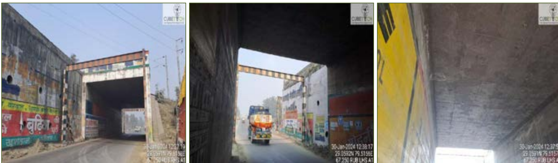
Figure 4-4: Condition of RUB
