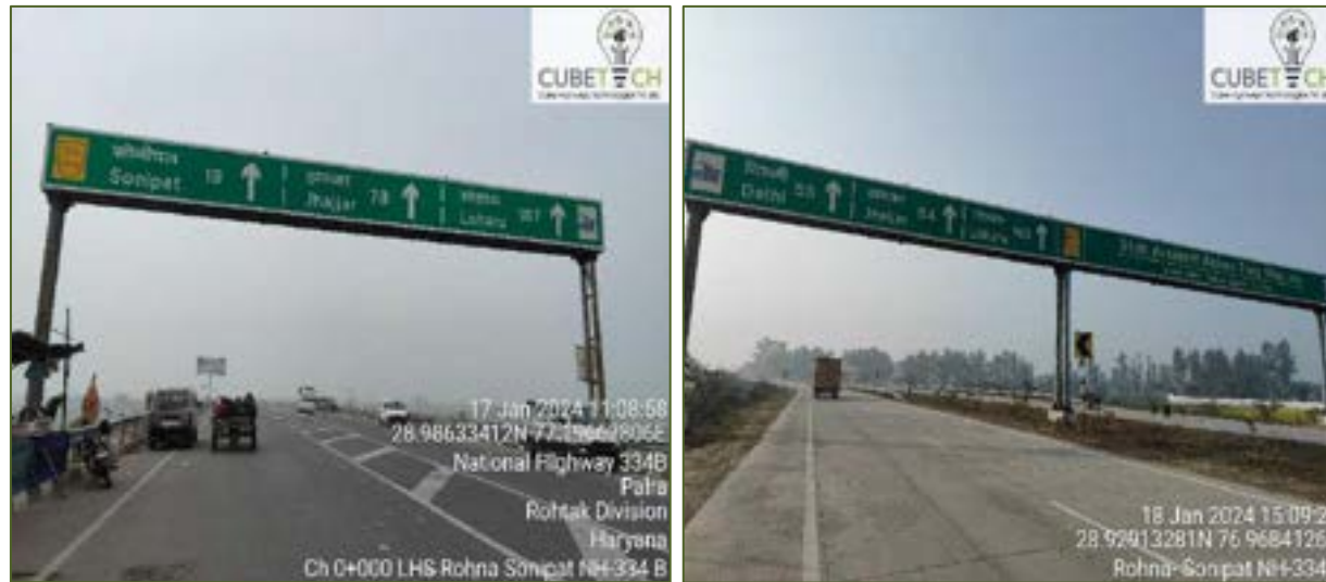
Figure 3-5: Overhead & Cantilever Gantry boards and VMS
